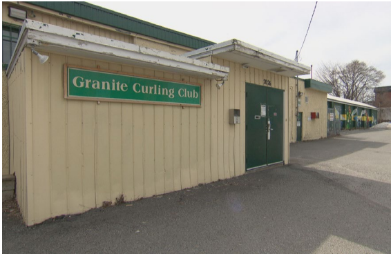
Figure 4.0 - Existing Granite Curling Club, 2026 Scott Street.
