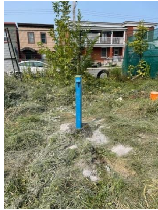
Conducting BH2 in restoration.
