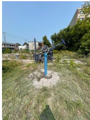
Conducting BH3 stick up on the subject property
