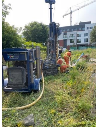
Conducting BH15 on what was once 249 Rochester Street.
