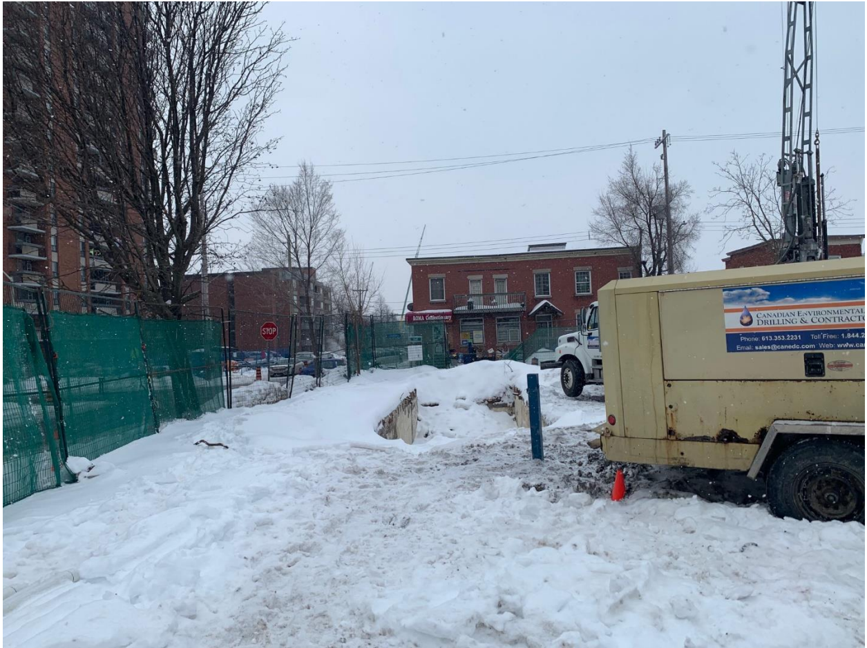
Image 1 – Monitoring Well 4, facing west (later decommissioned)
