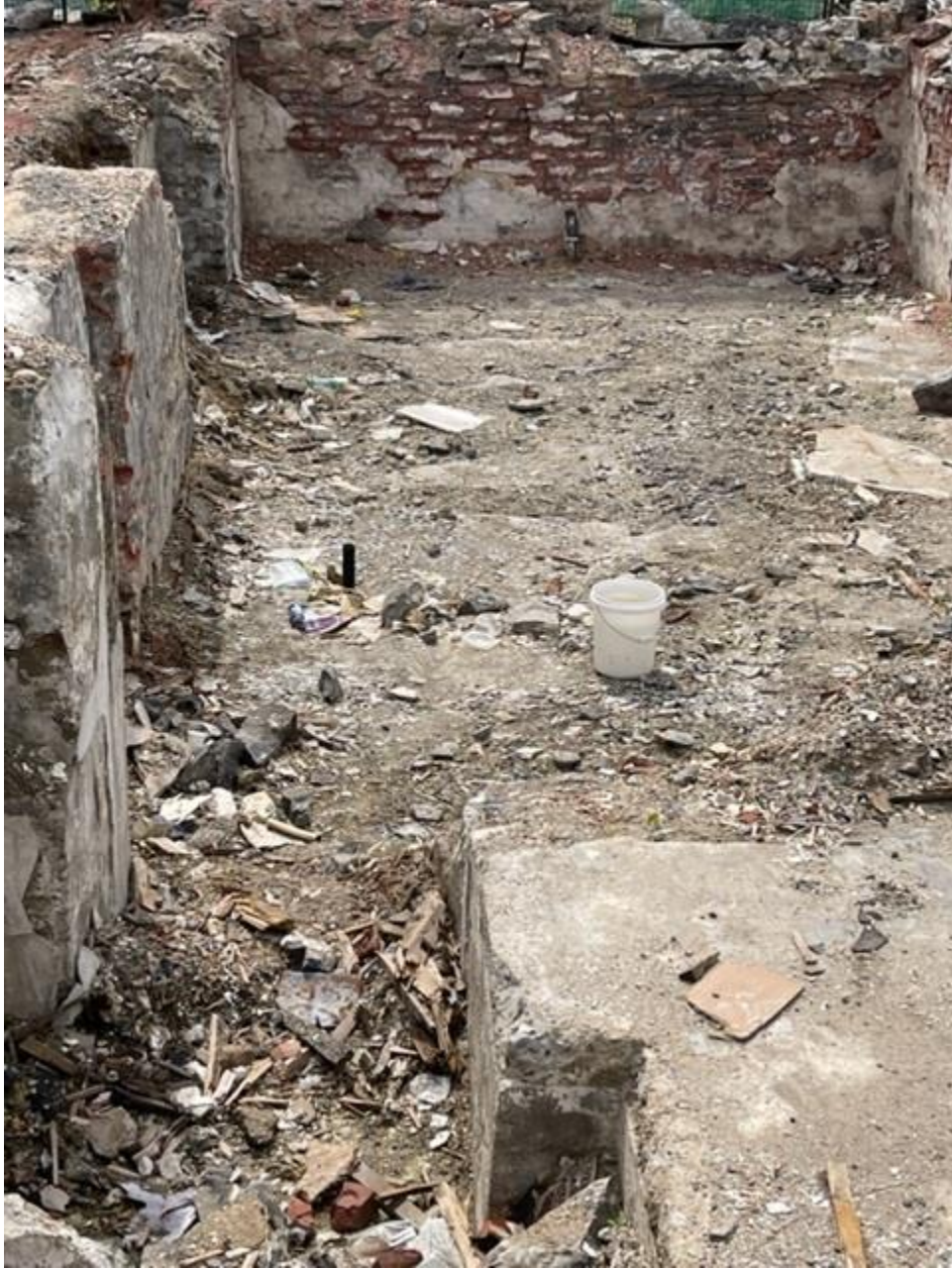
Image 3 - EXMW2 within the basement foundation
