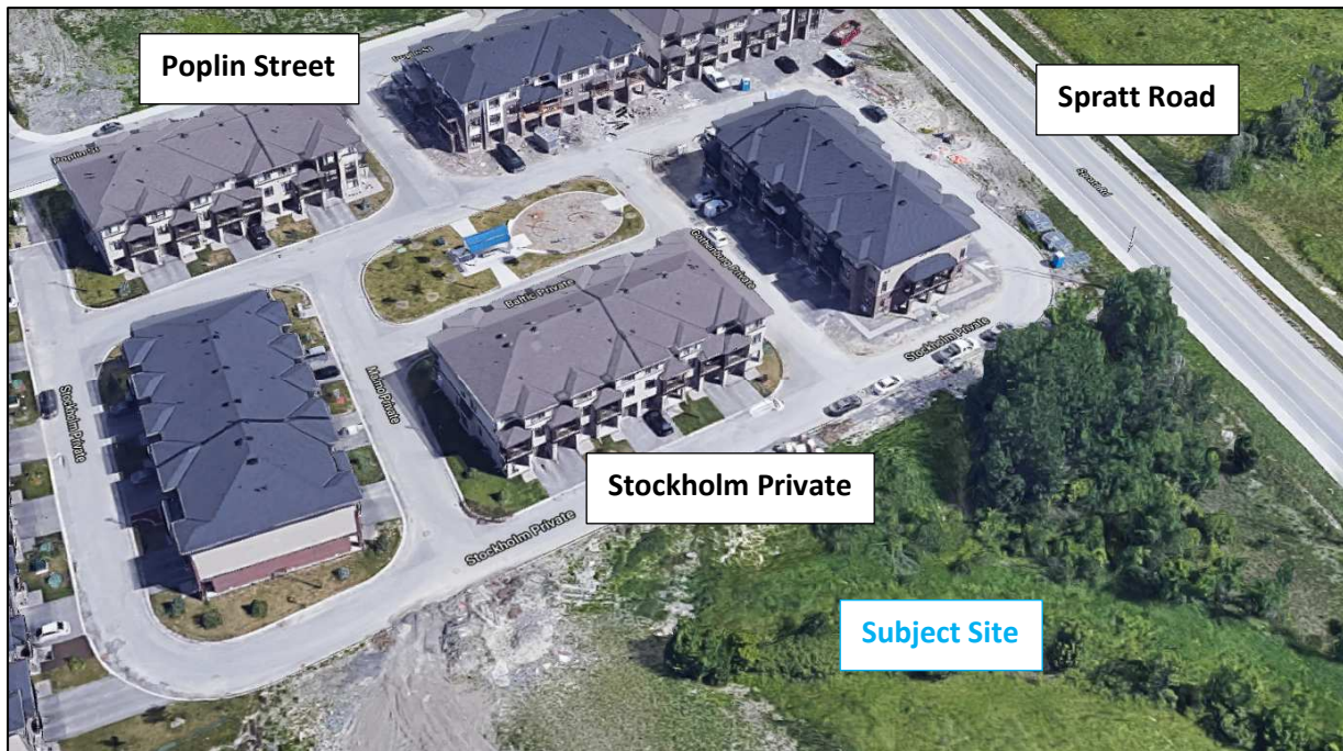
Figure 3: Looking north from above the Subject Site to the back to back townhouses to the north
