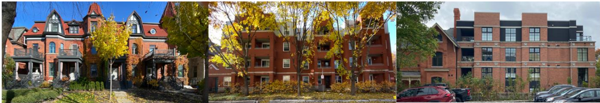
Figure 14: Examples such as Martin Terrace, King Edward Avenue, St. George's Coop Henderson Avenue, and Strathcona on the Park, Laurier Avenue illustrates the varied silhouette that incorporates a stepped profile at the upper floor.
