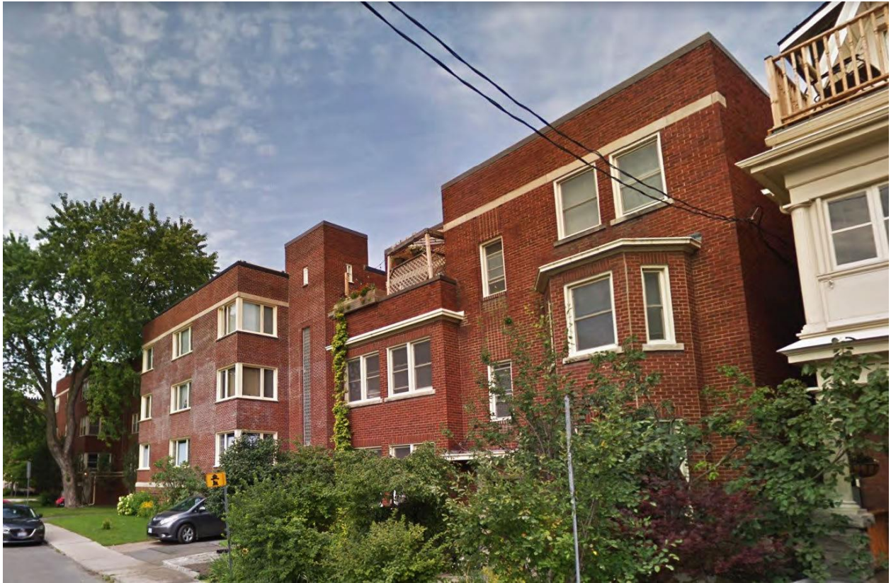
Figure 8: Street view of the apartment buildings at 175-179 Wilbrod and adjacent detached residence at 183 Wilbrod (right). Note the strong horizontal lines and asymmetrical massing of the apartment building. Source: Google Earth.
