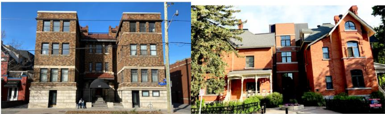
Figure 5: 165 Laurier Avenue and 417-421 Laurier Avenue are examples of “twin block” form found throughout the neighbourhood.
