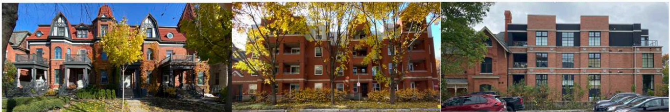
Martin Terrace, King Edward Ave St George's Coop Henderson Ave Strathcona on the Parc, Laurier Ave
