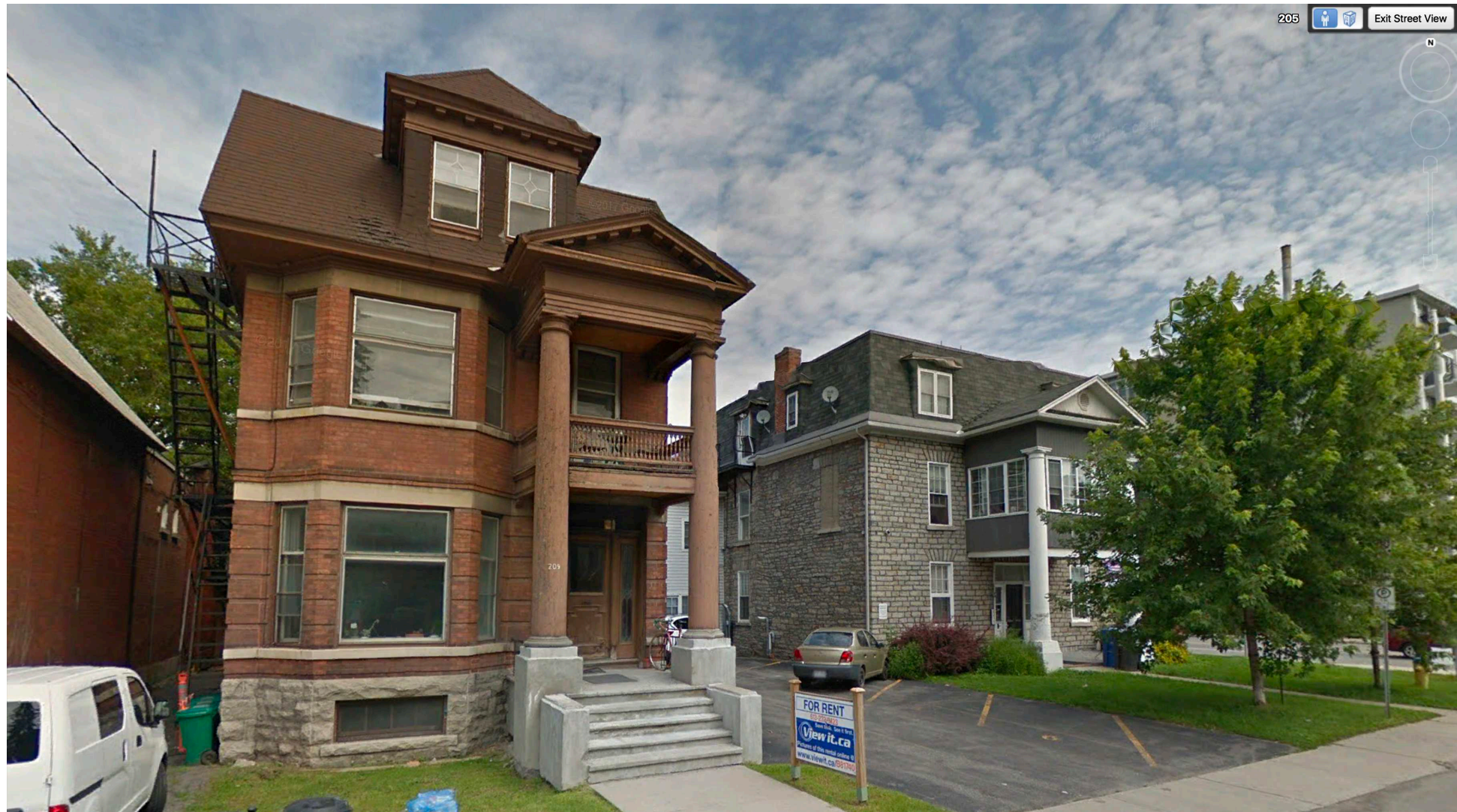
URBAN CONTEXT: WILBROD STREET (NORTH SIDE) LOOKING EAST TO KING EDWARD SHOWING 209, 211 WILBROD IN FOREGROUND
