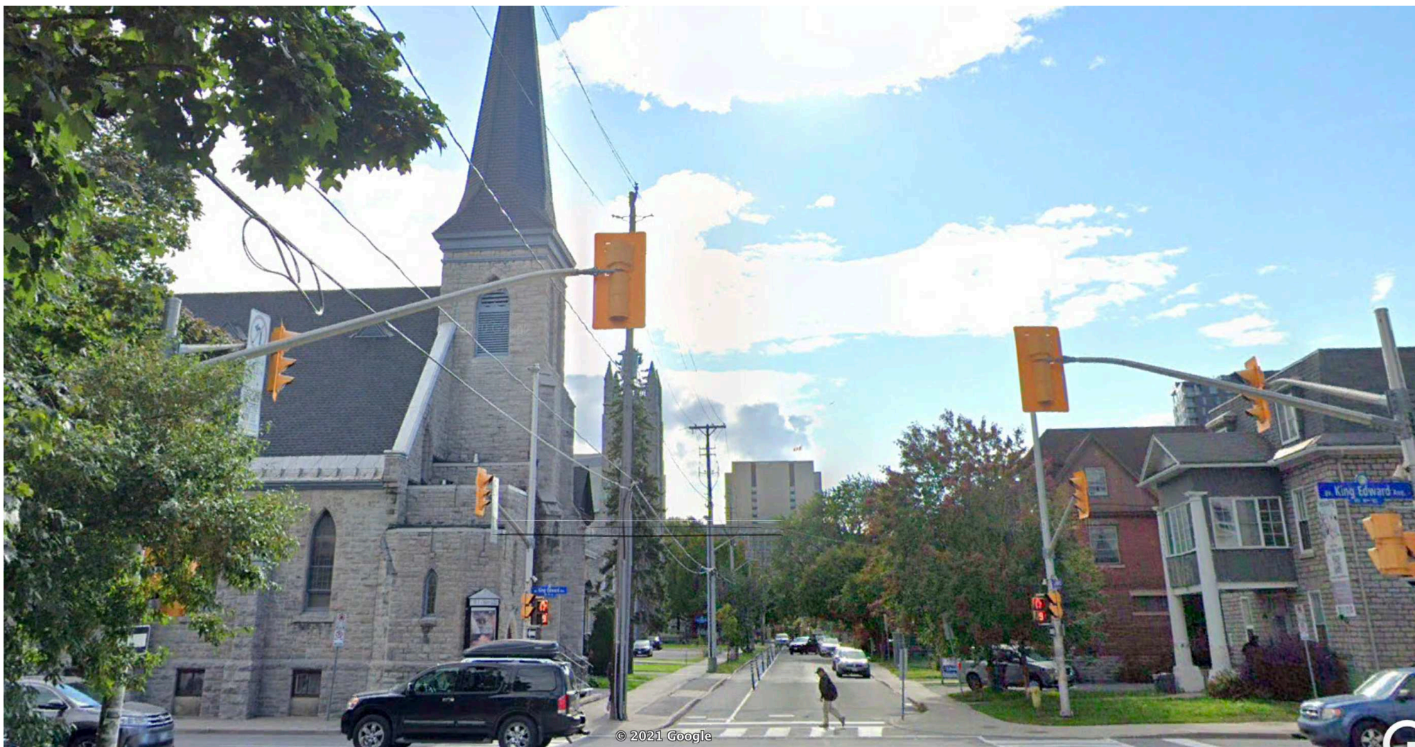
URBAN CONTEXT: WILBROD STREET LOOKING WEST FROM KING EDWARD AVE SHOWING ST PAUL'S LUTHERAN CHURCH IN FOREGROUND
