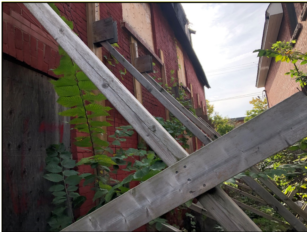
Photograph 4: View of the structural bracing erected on the east face of 197 Wilbrod Street, looking south.
