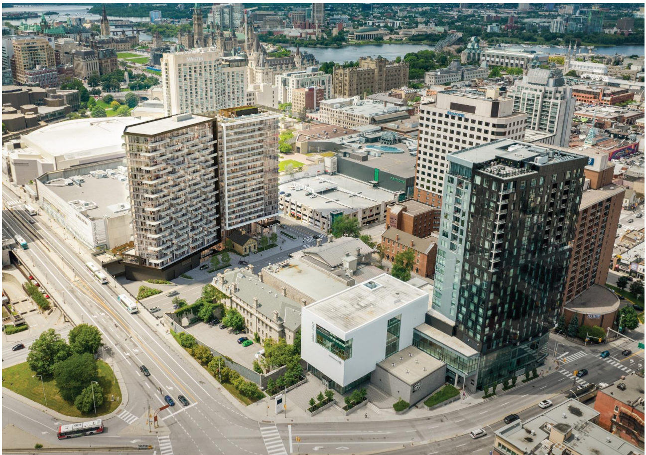
Figure 19: The aerial view provides the context for the development next to the Mackenzie King Bridge with the Rideau Centre in the background and the Arts Court across the street. Source: Zeidler, 2021.
