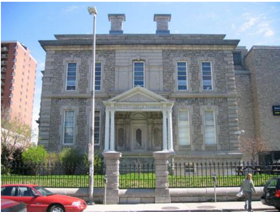
Figure 8: Carleton County Courthouse Nicholas Street façade. Note the masonry and metal perimeter wall/fence. Source: B. Padolsky Associates Inc. 2013
