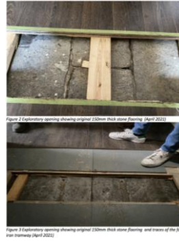
Figure 3 Exploratory opening showing original 220mm thick stone flooring and traces of the former tramway (April 2021)
