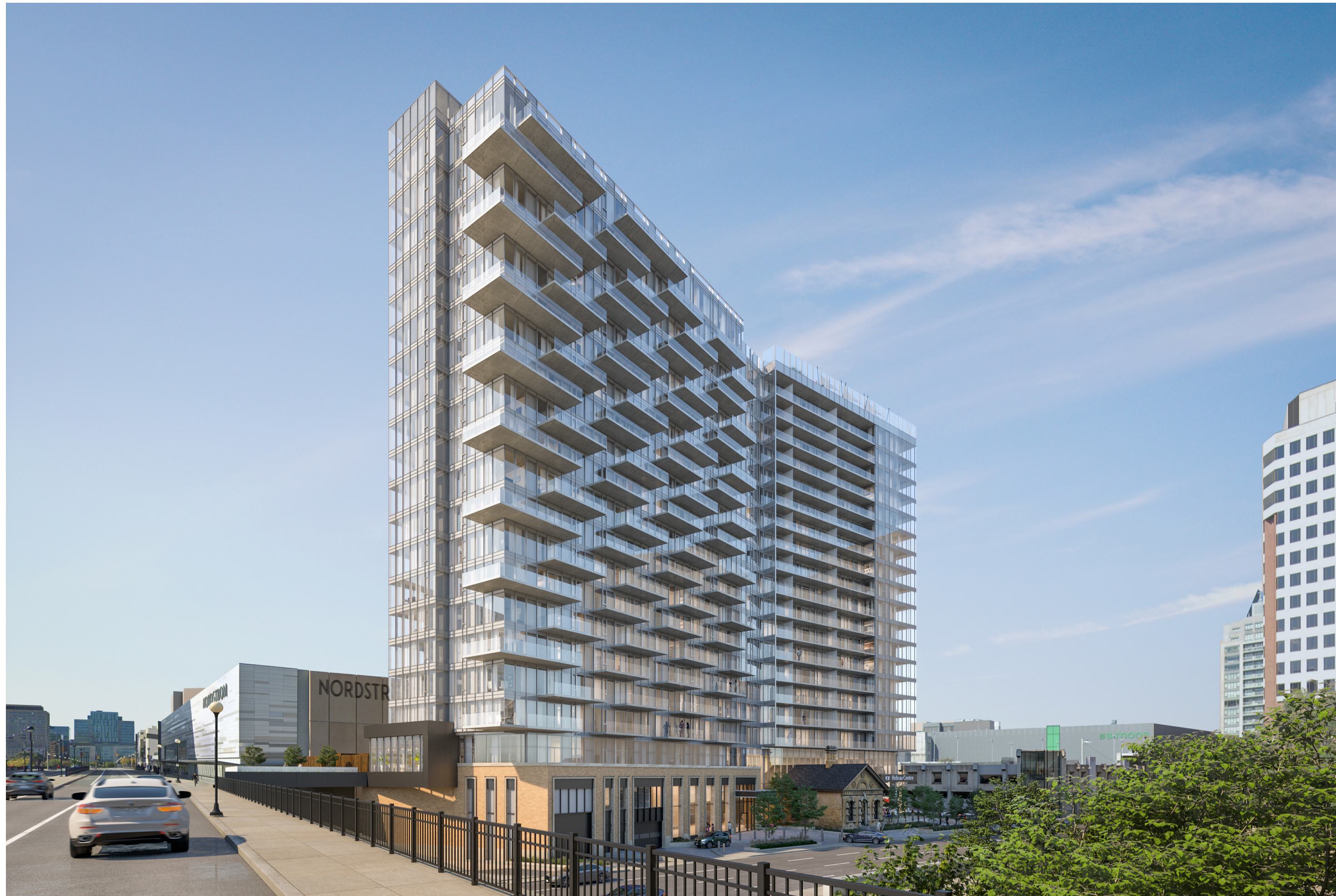
VIEW FROM SOUTHEAST ON MACKENZIE KING BRIDGE
