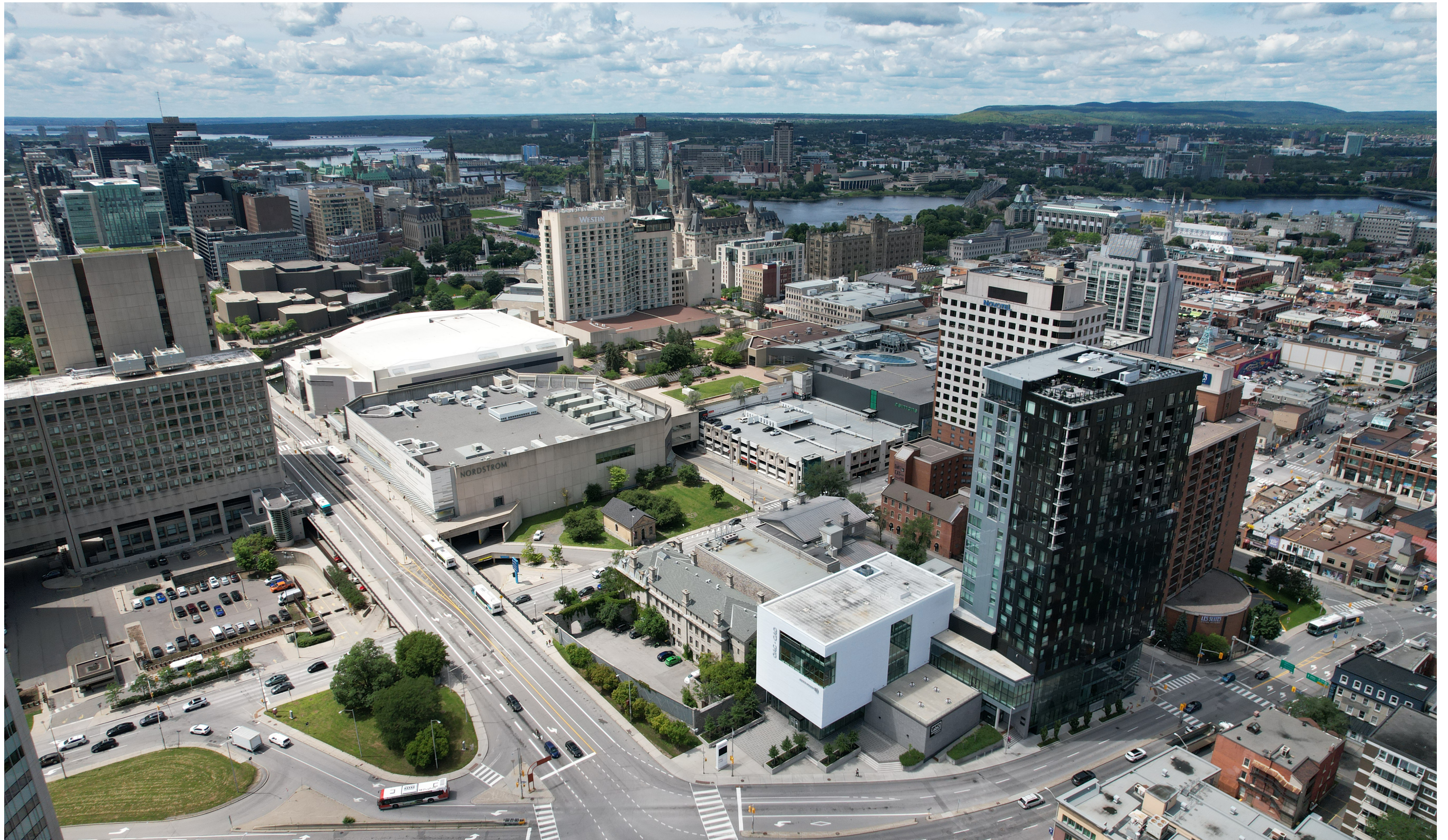
View from Southeast towards Parliament Hill - Existing Condition
