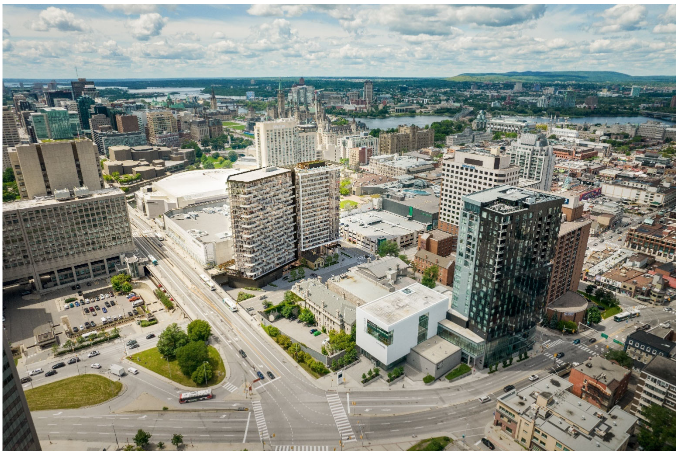
Figure 12: View Looking Northwest of the Proposed Development in Context
