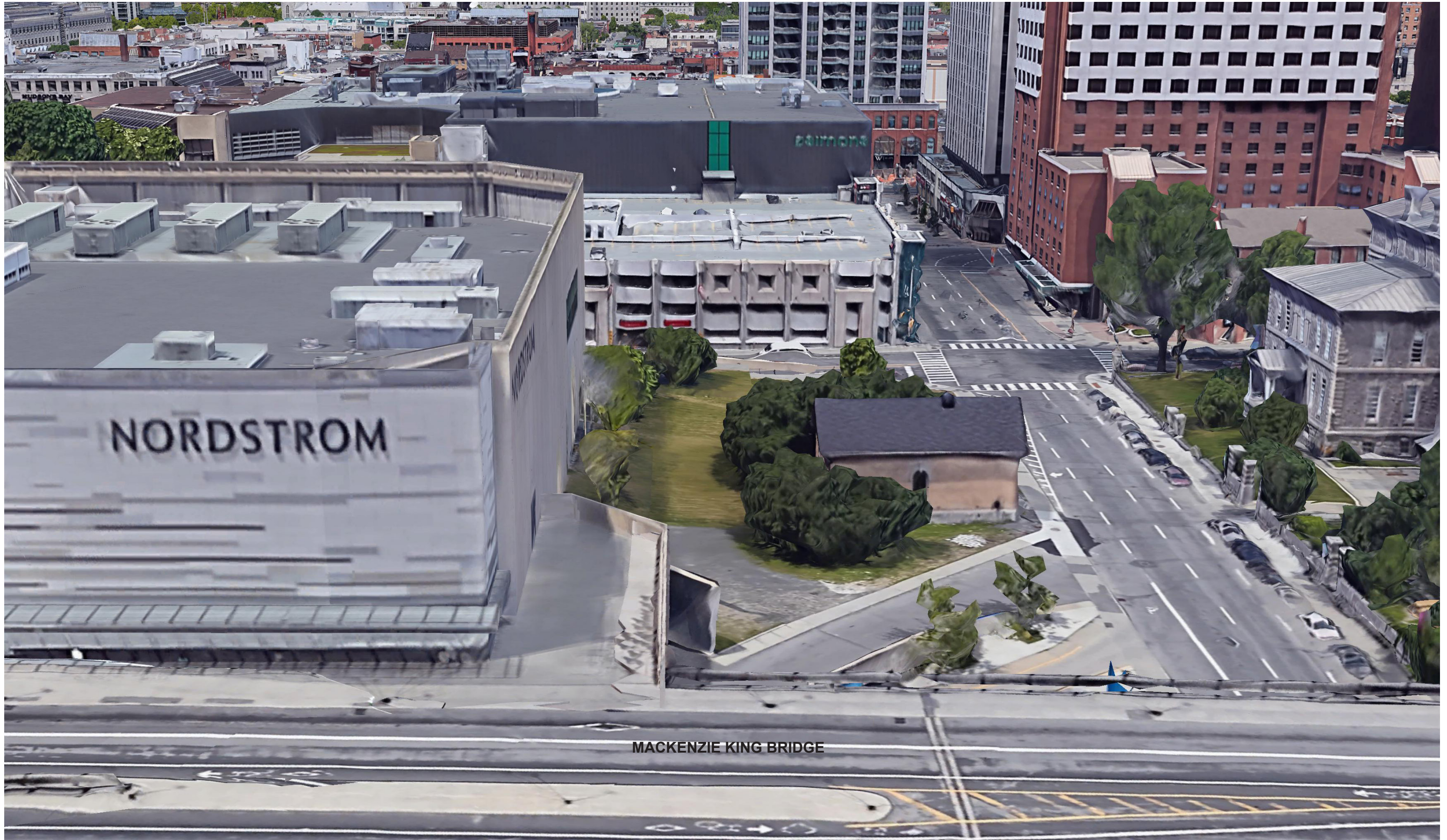
Mackenzie King Bridge Level - Existing Condition
