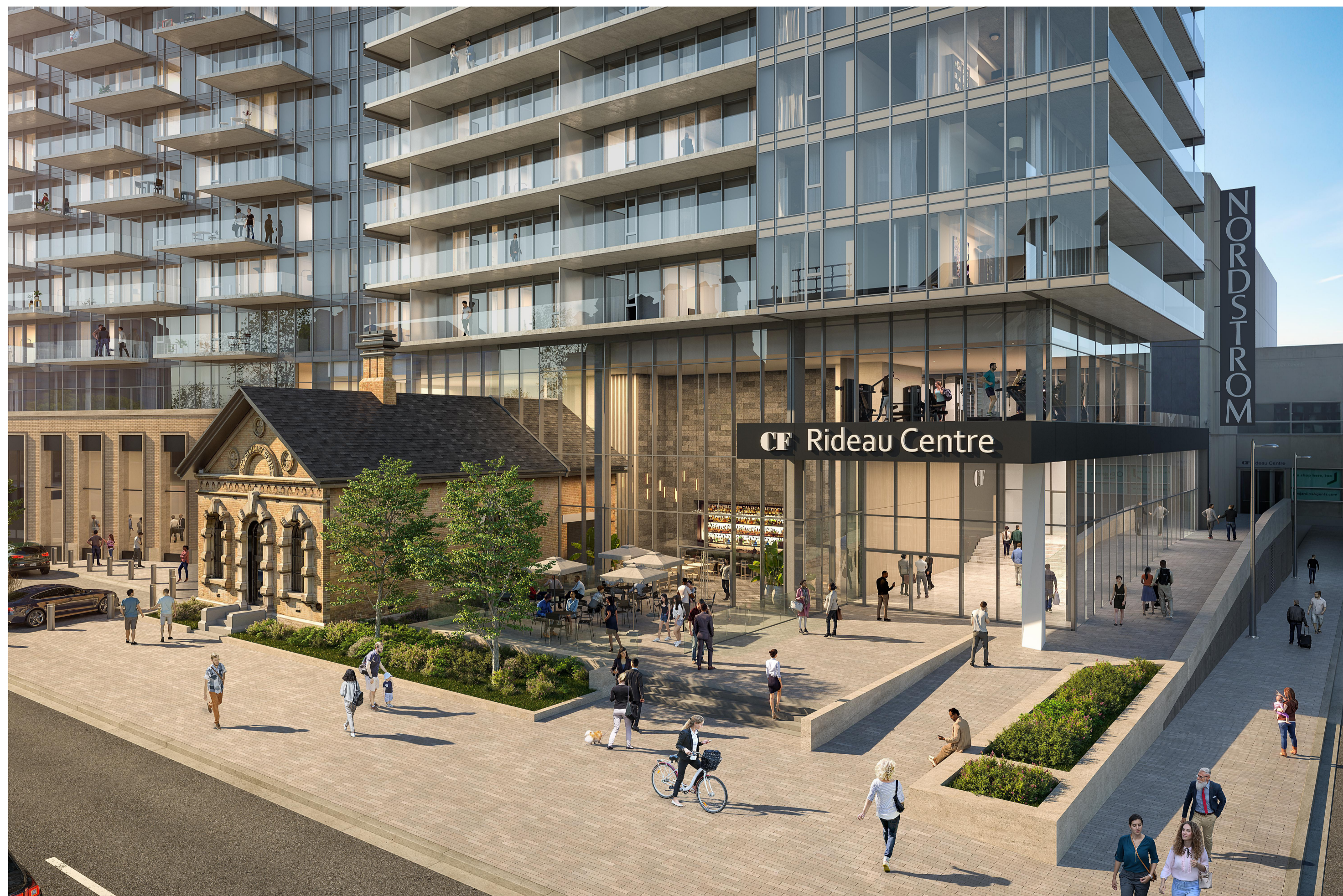
NORTHEAST VIEW FROM NICHOLAS ST
