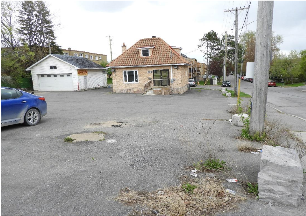
Photo 1: View of the Subject Property from the Northwest Corner Facing South. (May 7, 2021)
