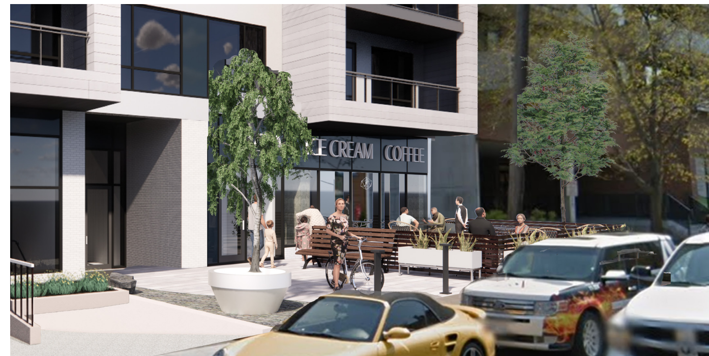
The north facade faces projects over the shared easement, by agreement between the property owners. Balconies face the front and rear of the property, with a central vertical band with a shifting interplay of grey and white panels for visual interest.
