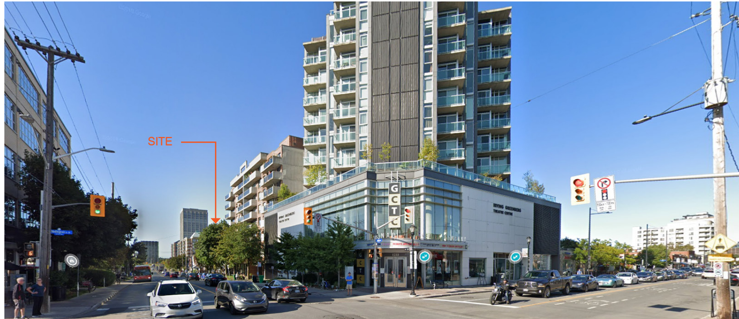
1 - VIEW FROM WELLINGTON ST W x HOLLAND AVE, LOOKING NORTH
