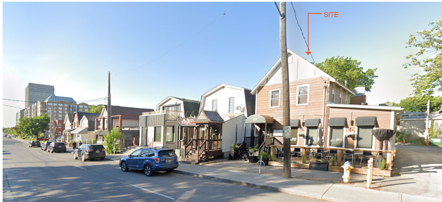
3 - VIEW FROM HOLLAND LOOKING NORTH AT SITE
