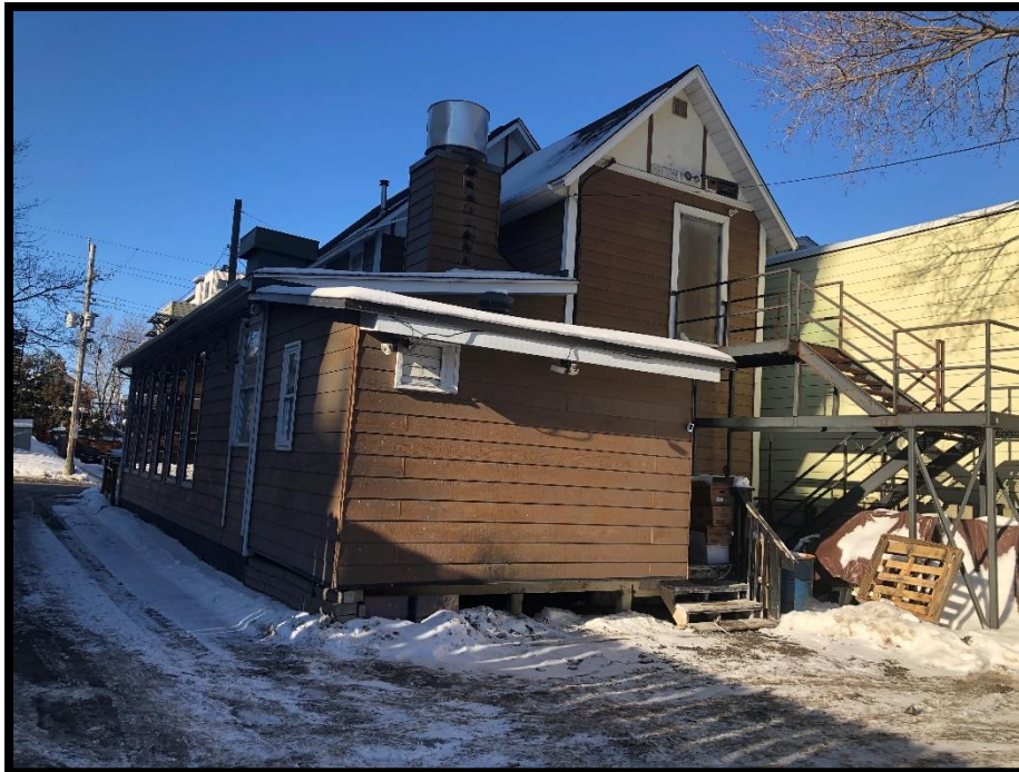
Photograph 2: Rear façade and addition of 93 Holland Avenue, facing west.
