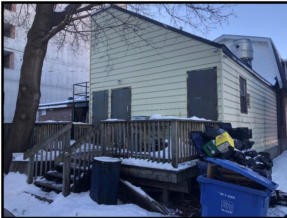
Photograph 6: Rear addition and waste bins of 91 Holland Avenue, facing west.
