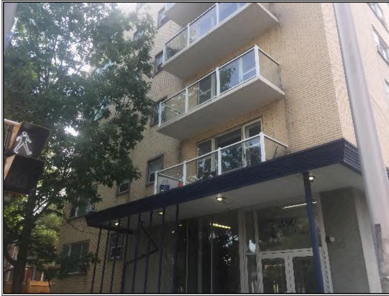
Photo 1 – Site Building (north elevation).
