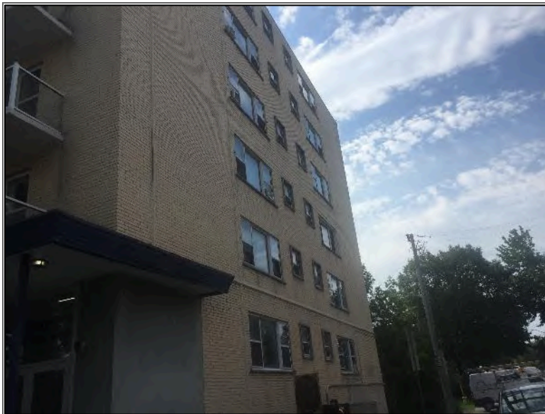
Photo 4 – Site Building (west elevation).
