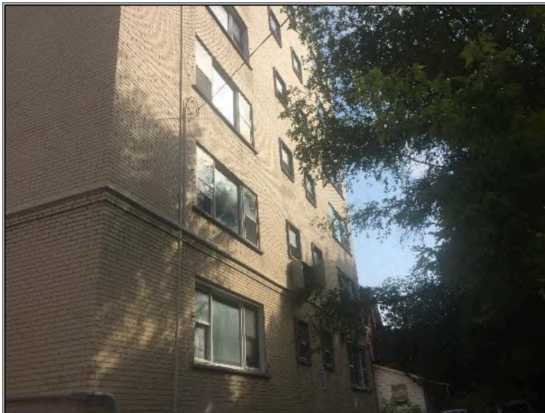
Photo 2 – Site Building (south elevation).
