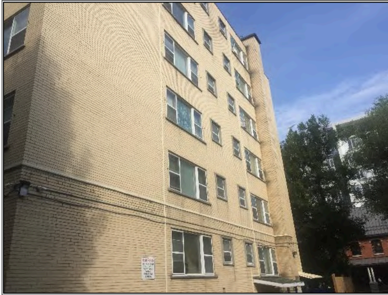
Photo 3 – Site Building (east elevation).
