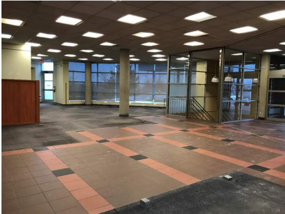
Photo 7 - Overview of the main level of the building
