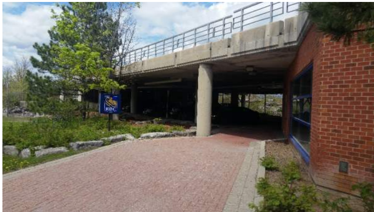
Photo 10 – First floor of the parking structure and Site building from west side of Site (facing northeast).
