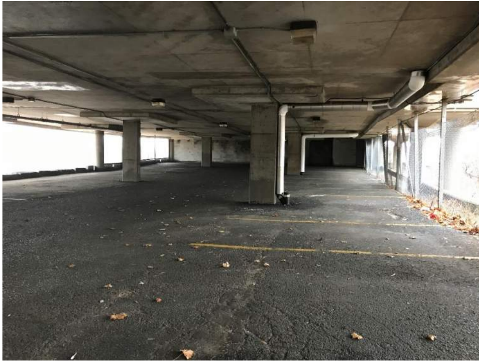
Photo 15 – View of the lower level of the parking garage
