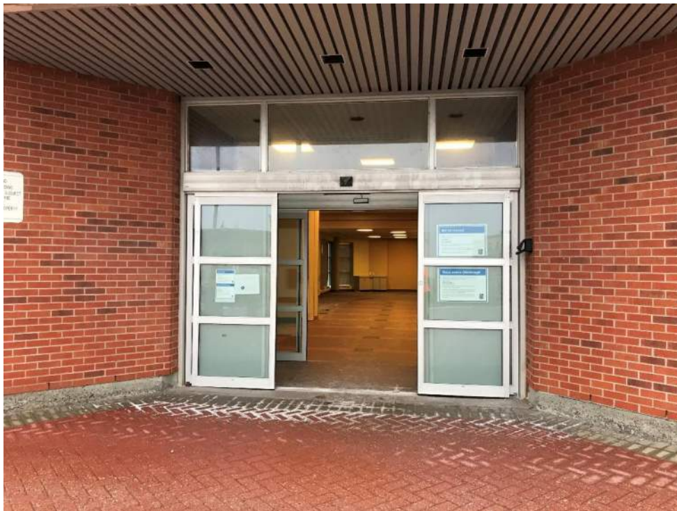
Photo 6 - View of the building's main entrance
