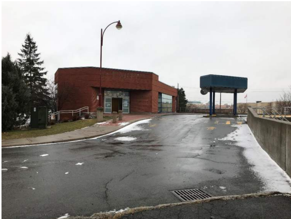
Photo 2 - View of the driveway to the upper level of the parking garage and the east side of the building
