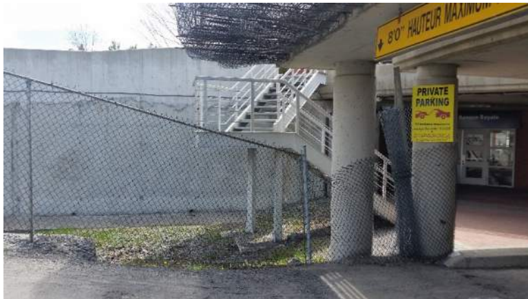
Photo 18 – First floor parking lot entrance to structure and RBC (facing south).
