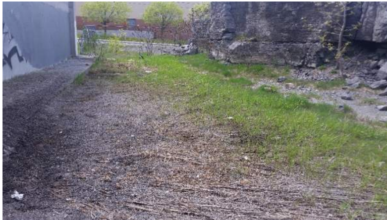
Photo 19 – South wall of the parking structure and exposed bedrock (facing west).
