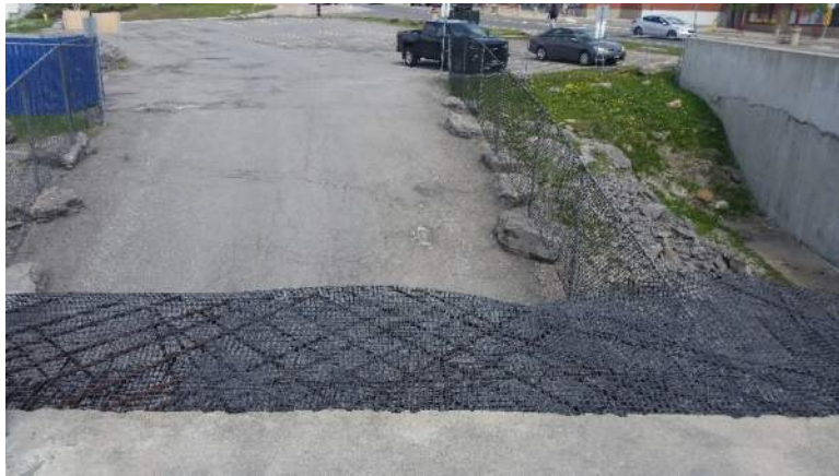
Photo 7 – Looking down from the second story of the parking garage to the first floor entrance (facing east).
