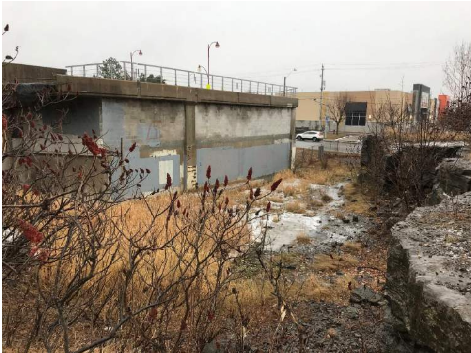
Photo 22 - View of the northern exterior wall of the parking garage and the rock wall surrounding the garage
