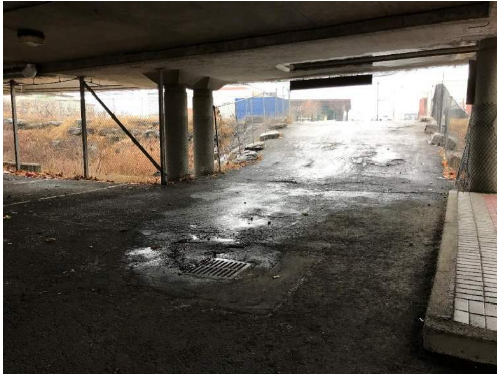
Photo 17 - View of the parking garage entrance ramp, facing east
