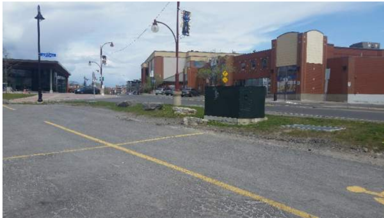
Photo 5 – Site parking lot, transformer, Centrum Boulevard, commercial properties and Shenkman Arts (facing southeast).
