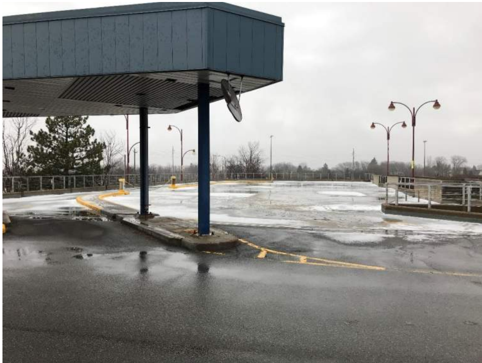
Photo 4 – Overview of the upper level of the parking garage
