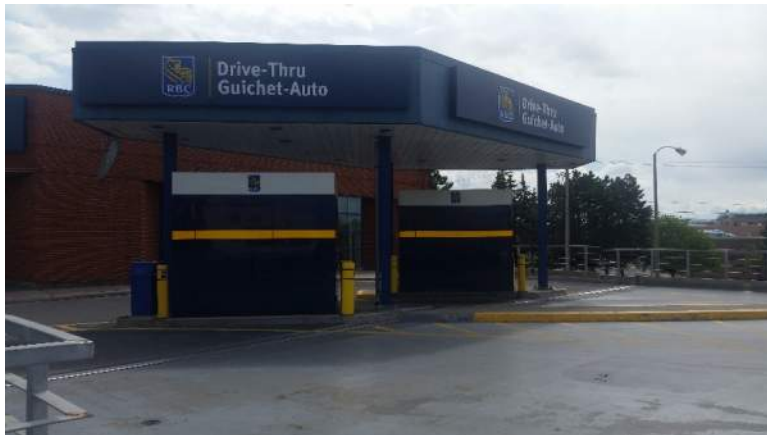
Photo 6 – Site building RBC drive-thru on the second floor of the parking garage (facing west).
