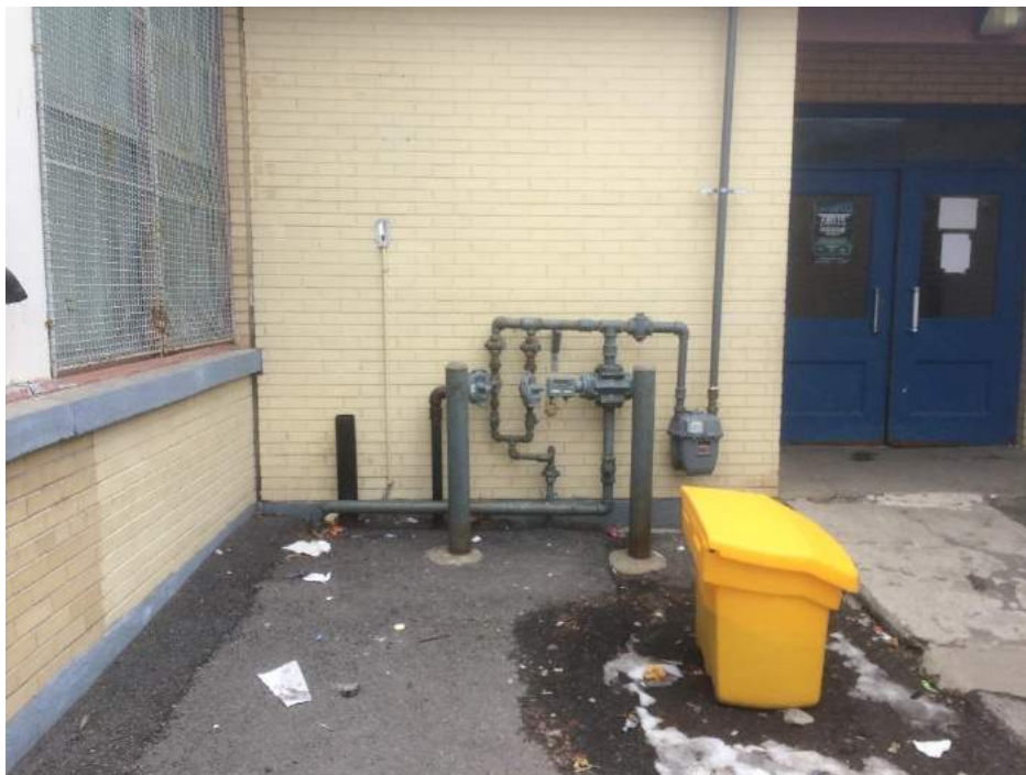
Photograph 2: Natural gas connection for the subject site and vent and fill pipes.
