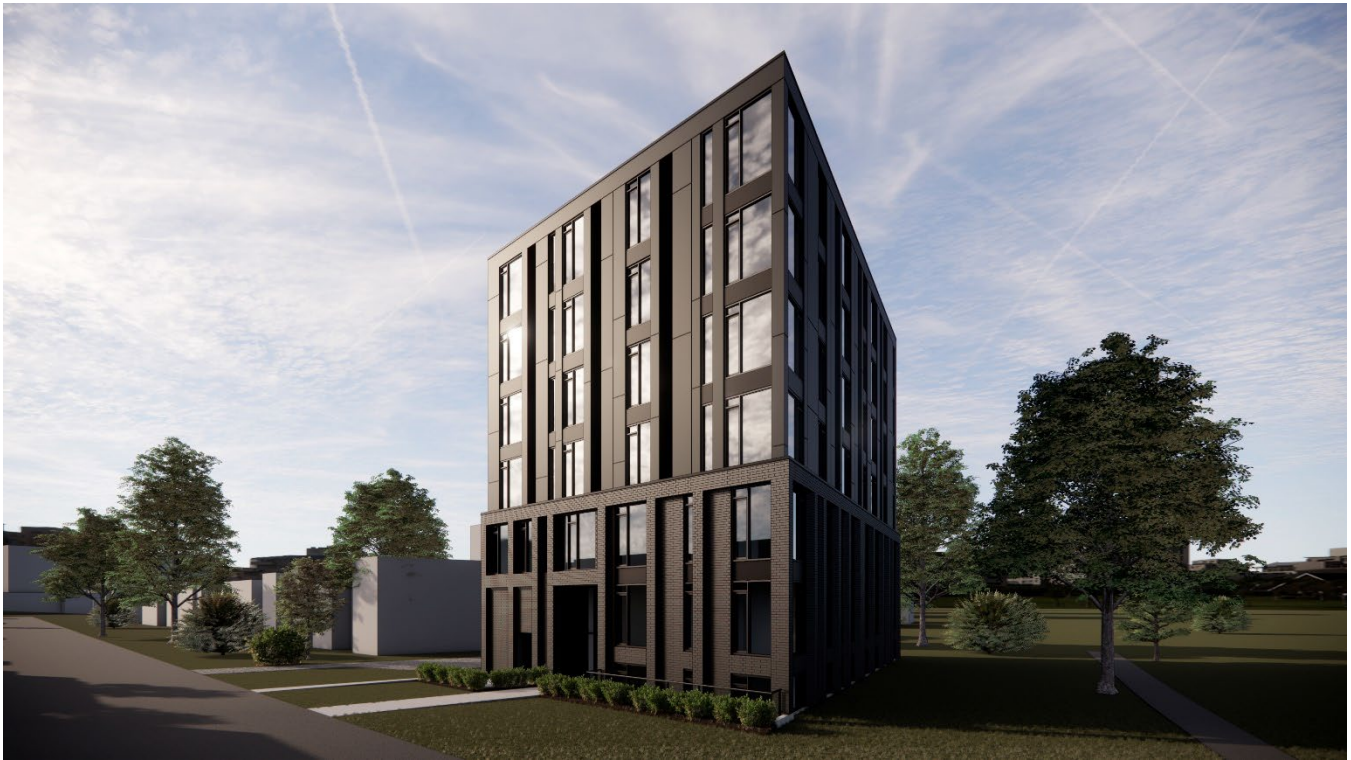
Figure 6: Excerpt from the site plan of the proposed development at 342 Roosevelt Avenue
