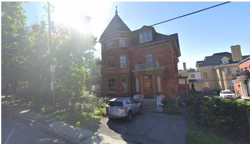
Figure 3 – View of the current building at 320 Chapel Street
