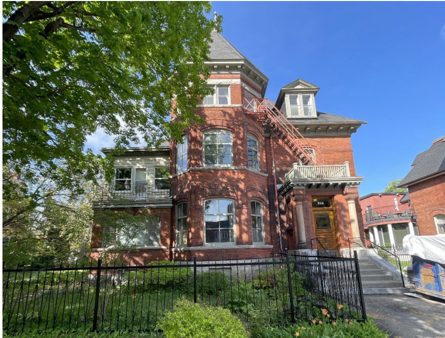
Photo 1 View of the east portion of Site Building A, May 20, 2026.
