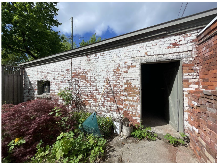
Photo 4 View of the east portion of Site Building B, May 20, 2026.
