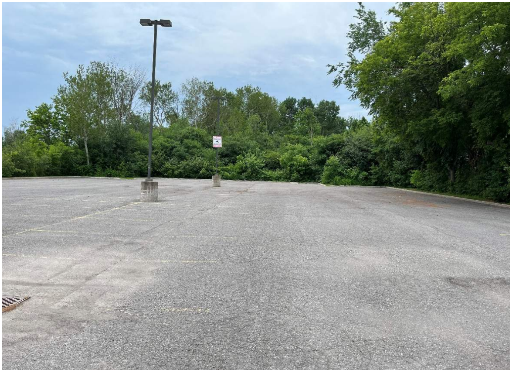
Photograph 6: View looking south from the south side of the subject building.
