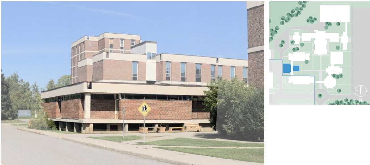
Figure 8. Building I viewed from southwest (ERA, 2021).
