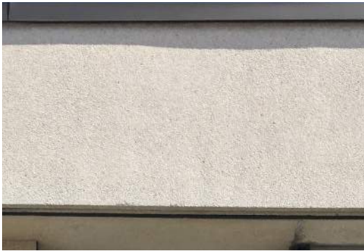
Figure 23. Aggregate-faced concrete paneling (ERA, 2021).
