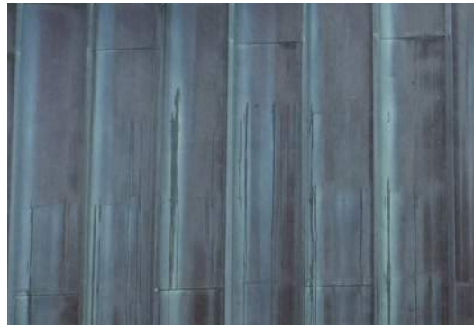
Figure 22. Standing seam copper roofing (ERA, 2021).
