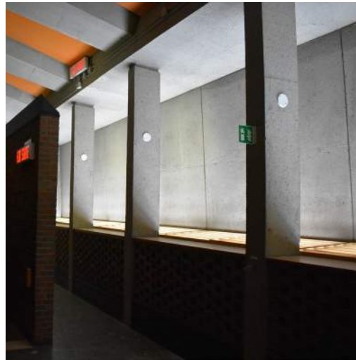
Figure 18. Building A, columns and water detail (ERA, 2021).
