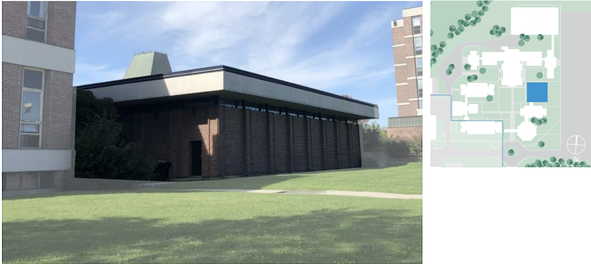
Figure 5. Building D, viewed from southeast (ERA, 2021).
