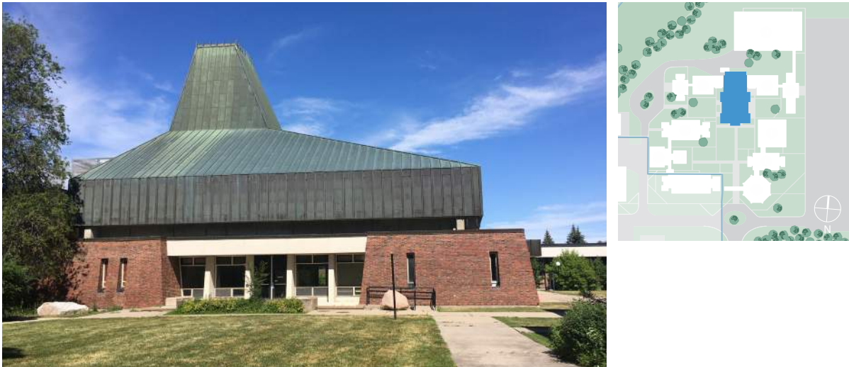
Figure 2. Building A, west elevation (ERA, 2021).
