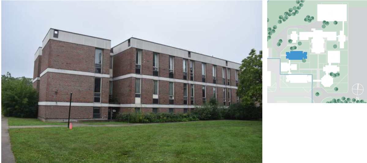
Figure 9. Building J, from Sisters' courtyard (ERA, 2021).
