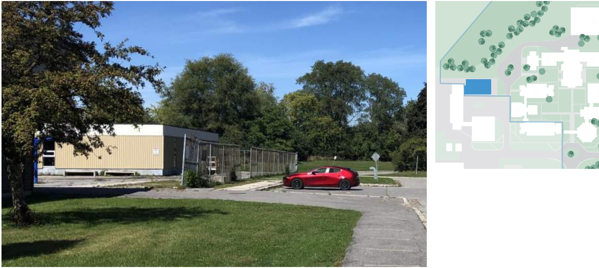
Figure 11. Building N, viewed from south-east (ERA, 2021).
