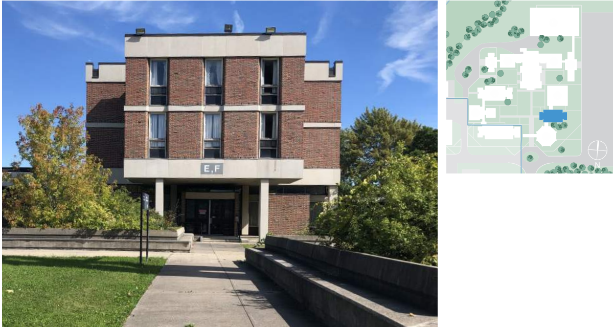
Figure 6. Building E, west elevation (ERA, 2021).
