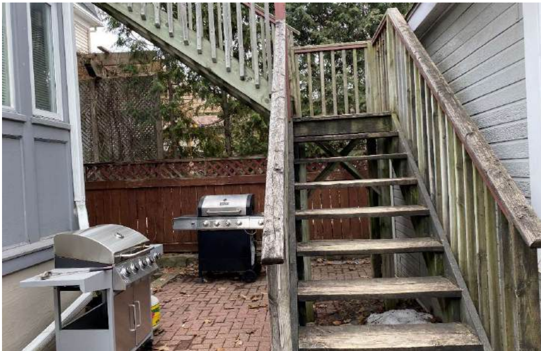
Photograph 4: View of rear patio.
