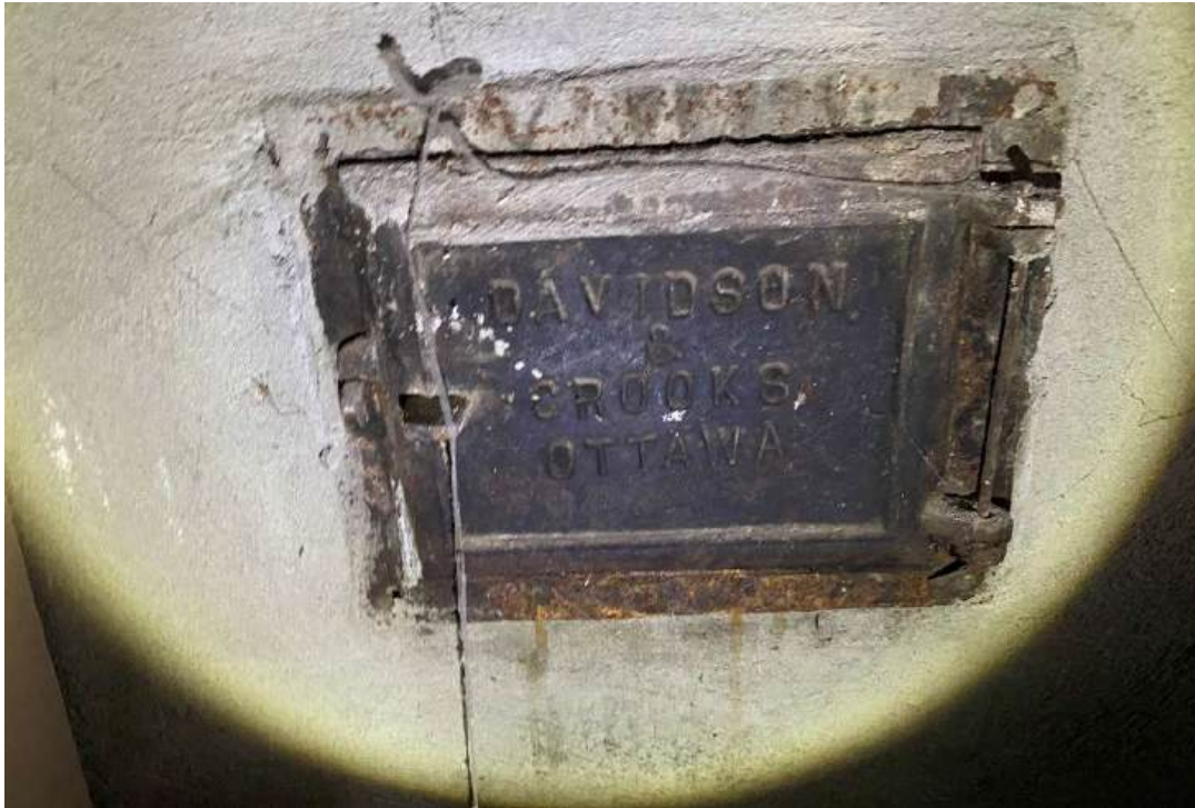
Photograph 3: Chimney cleanout in basement.
