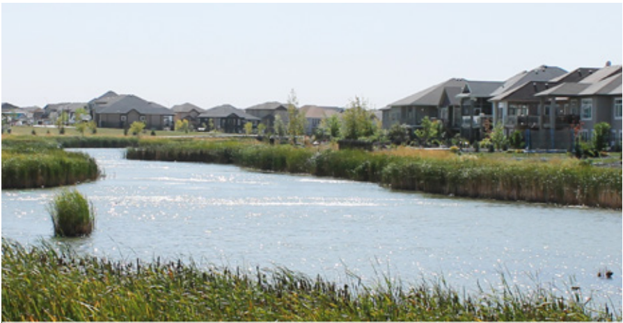
Stormwater Management Pond
