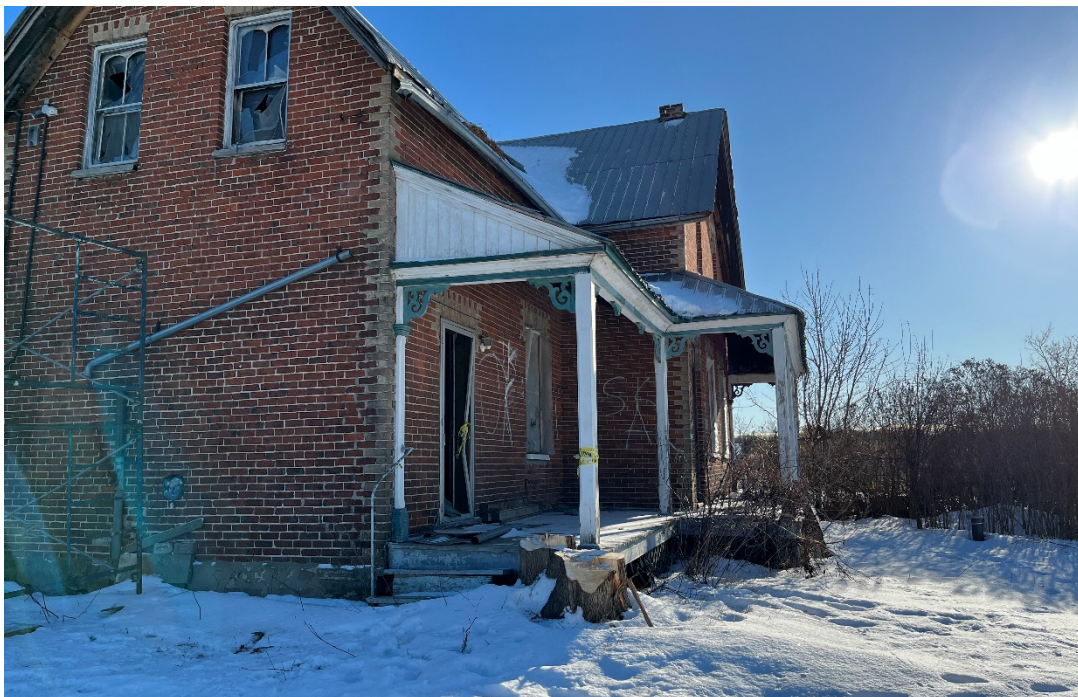
Photograph 2: View of vacant residential dwelling in the north central portion of the Phase I Property.
