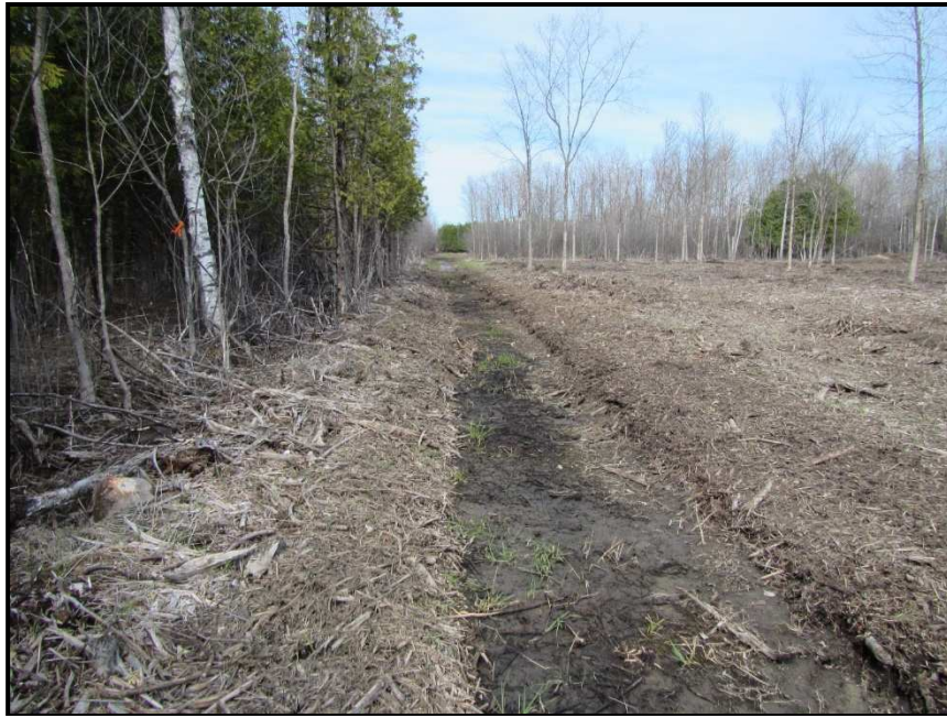
Photo 17 – Realigned dry northwest swale (April 29 th , 2016) along the north edge of the site. View looking east, with areas of tree cutting to the right, south, and MTO lands to the left, north
