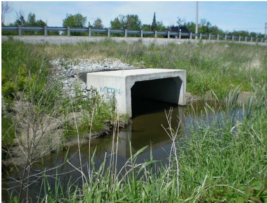
Photo 13 - Feedmill Creek as it enters the box culvert under Highway 417 north of the MTO lands. View looking downstream, northeast (June 10 th , 2016)
