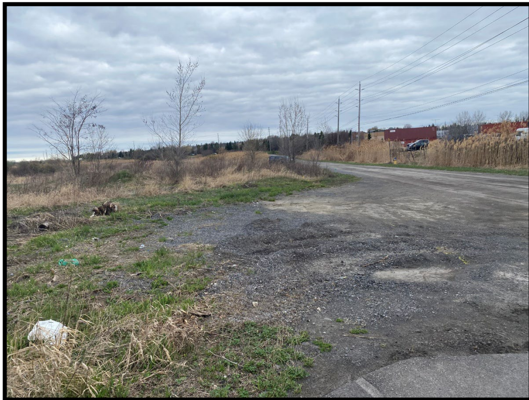
Figure 16: Example of disturbed conditions (MH1446-D062).
