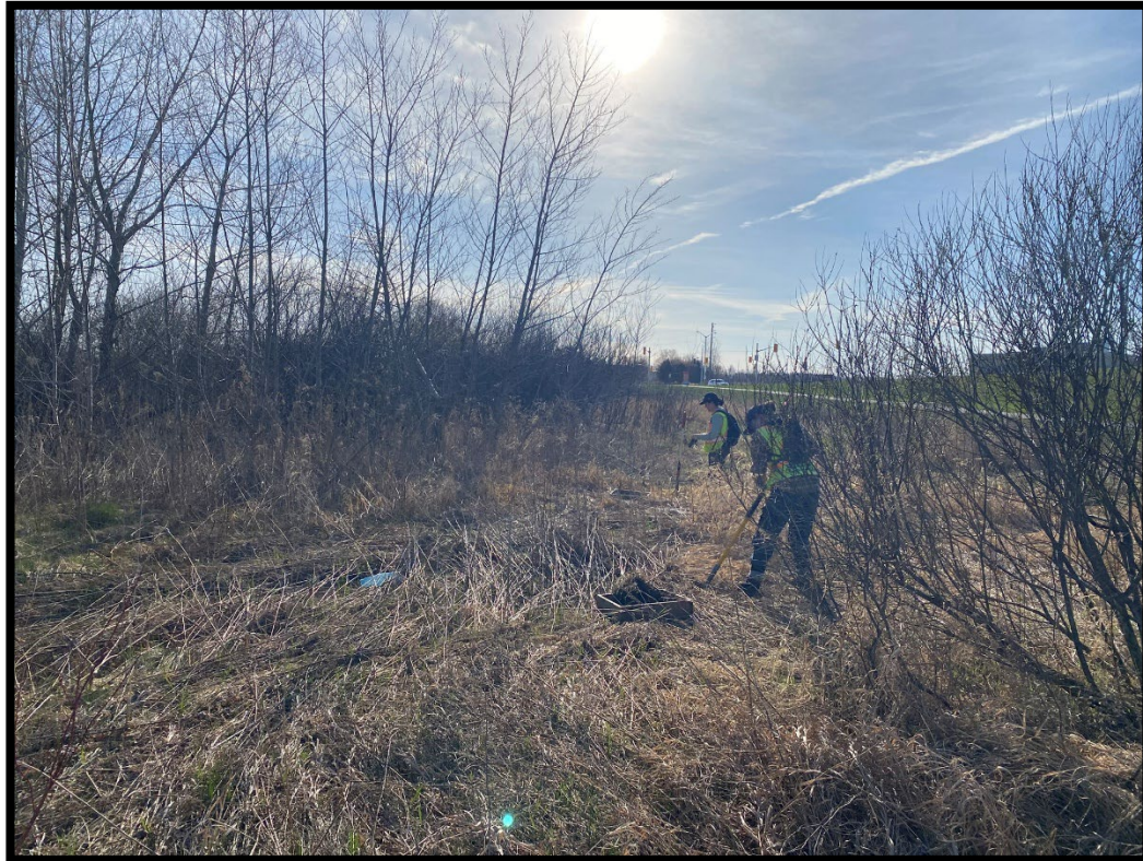
Figure 21: Test pitting in progress (MH1446-D002).
