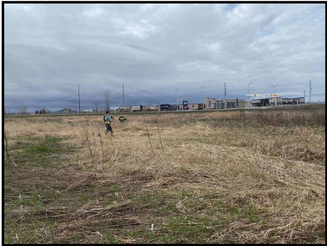
Figure 24: Test pitting in progress (MH1446-D067).
