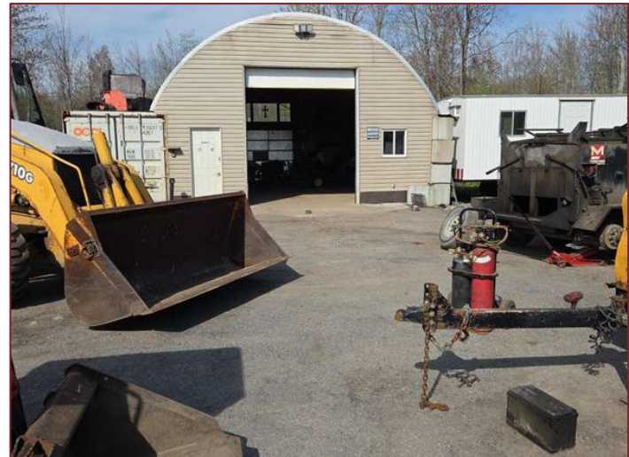
Photograph K8 – Looking west at small shop and adjacent office structure.
