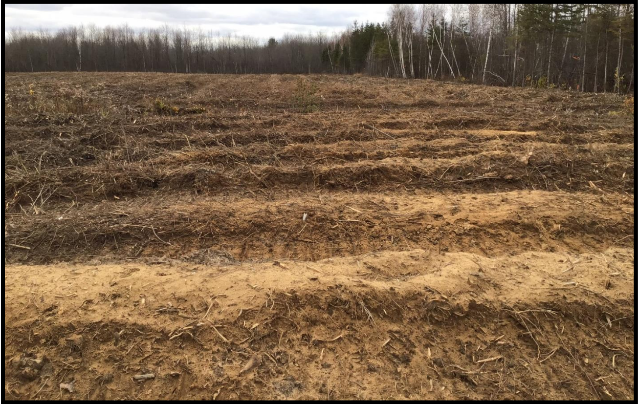
Figure 13: Extensive disturbance from grubbing in central-southern portion of study area. Note subsoil exposure. (PA1164-D12)
