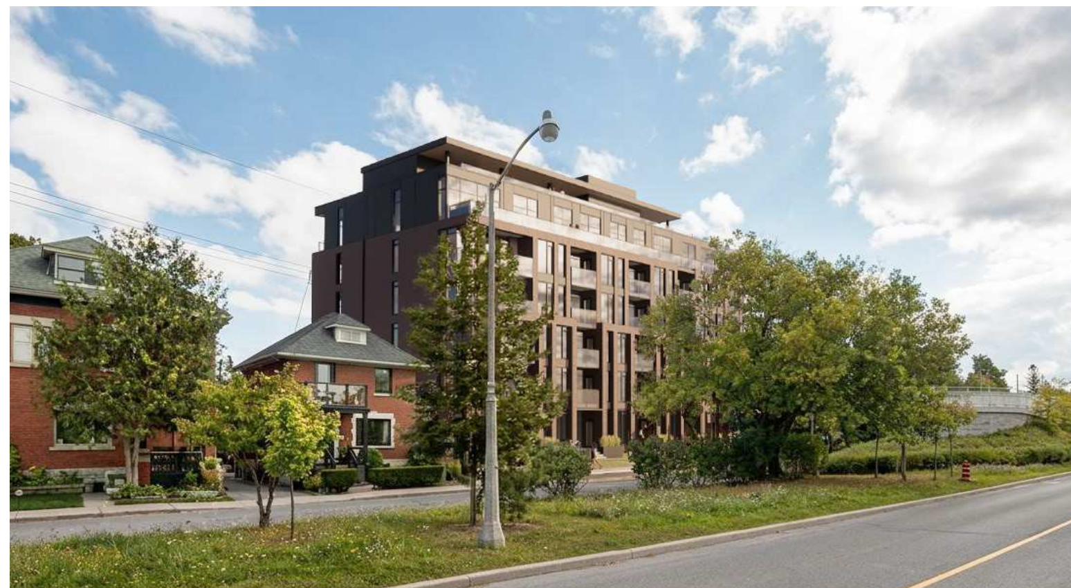
View From Colonel By Drive Looking South-East
