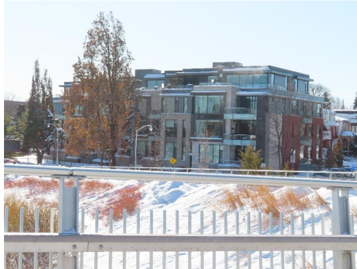
Figure 11: Residential building located on the opposing side of the Flora Footbridge, featuring similar materiality and adjacencies to the canal (Source: Juxta Architects).
