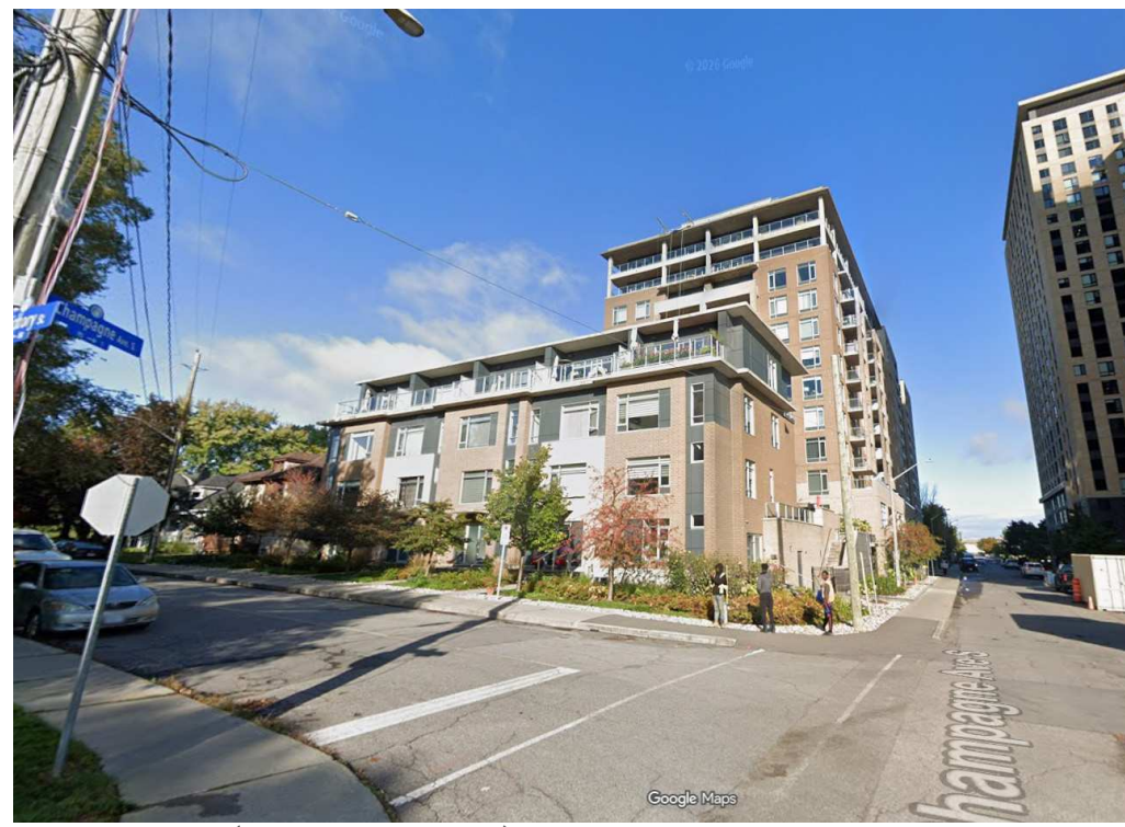
3. Hickory St. (View North-West)
