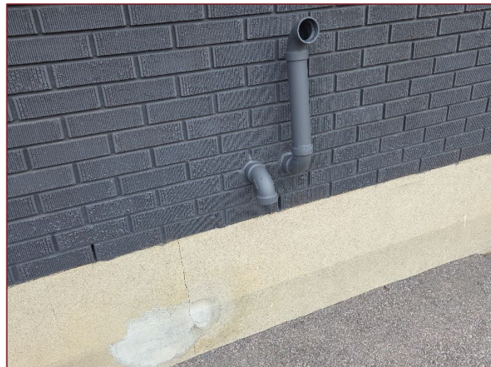
Photograph K14 – Looking east at the side of the residential building with a historic fill and vent pipe for the historic UST.
