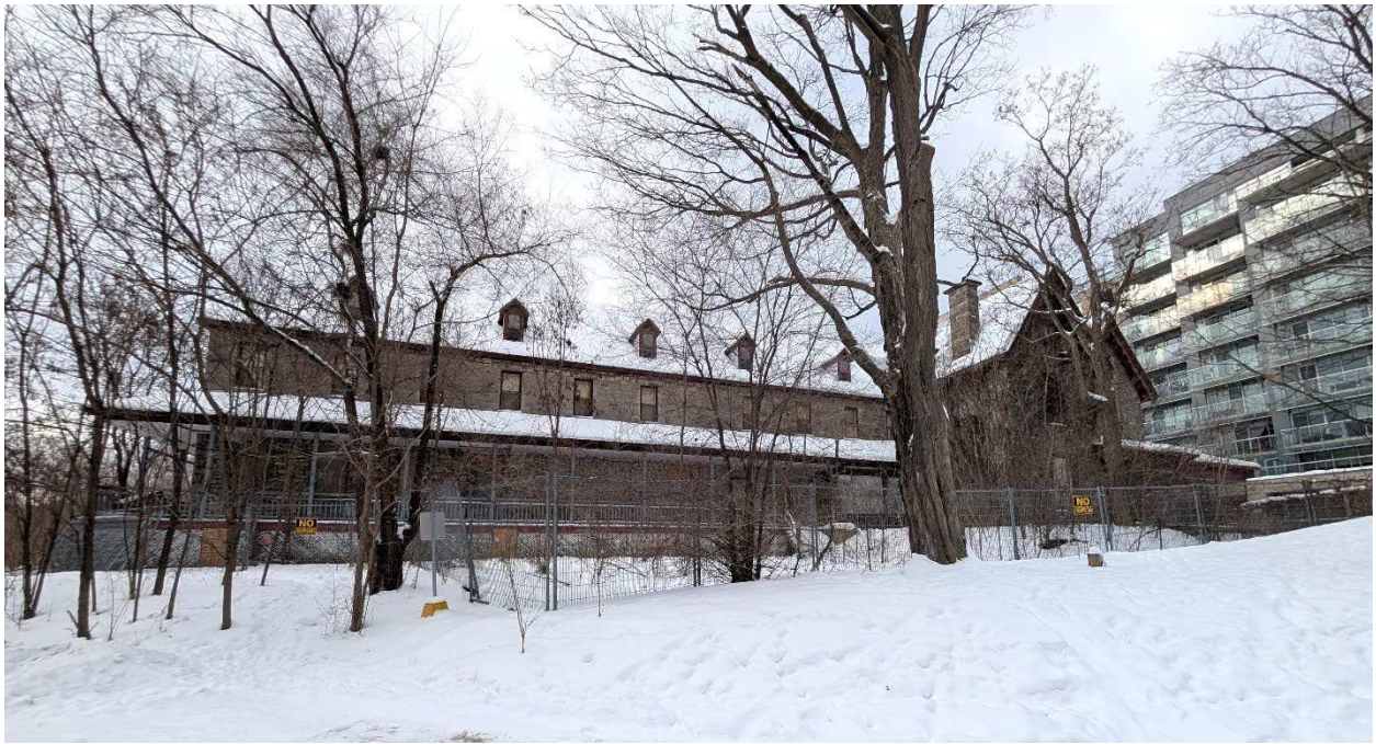
Figure 7: East elevation of the east wing and Gothic Revival house. (Heritage Studio, January 2026)
