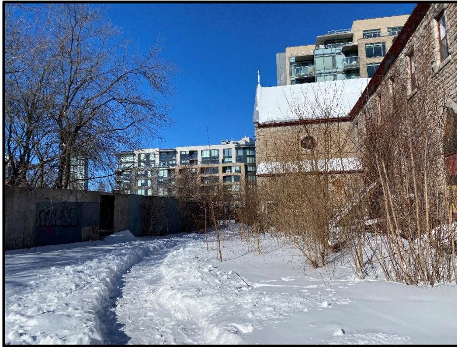
Photo 1: West side of the subject building facing north.
