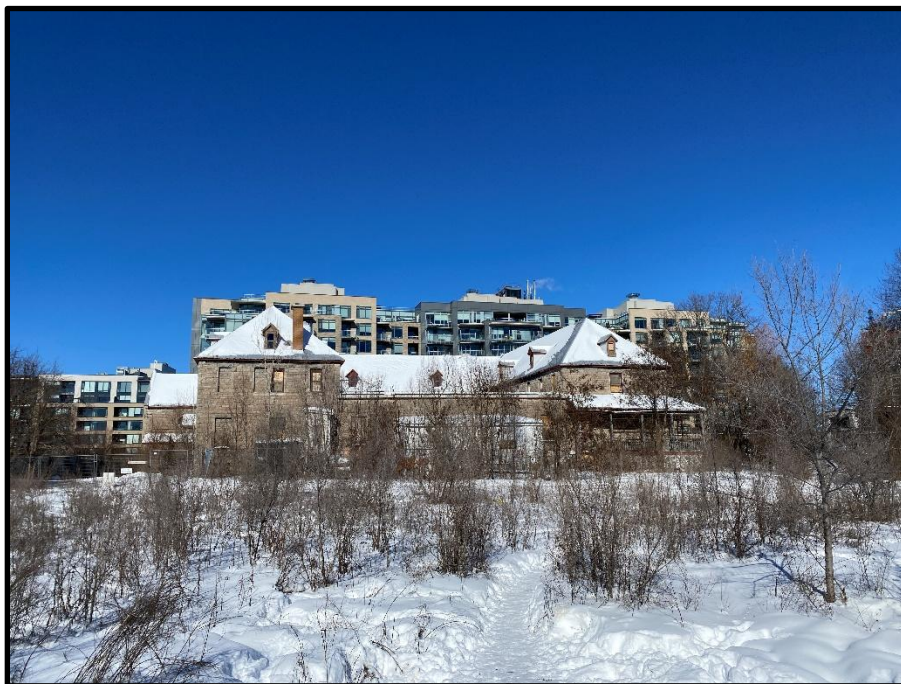
Photo 6: South side of the subject building facing north.
