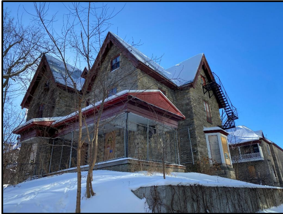
Photo 3: North east corner of the subject building.
