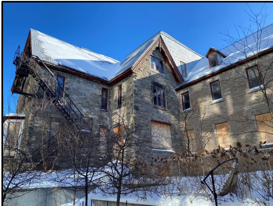
Photo 2: North side of the subject building.
