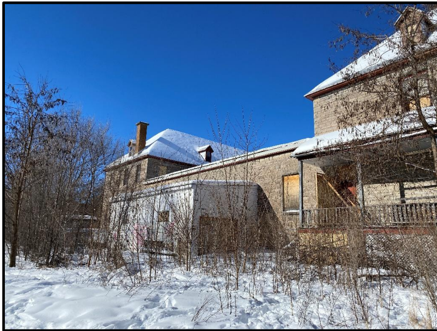
Photo 5: South side of the subject building.
