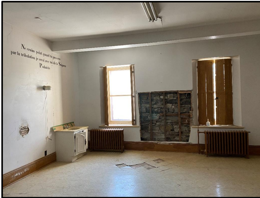
Photo 13: Room on second floor of subject building.
