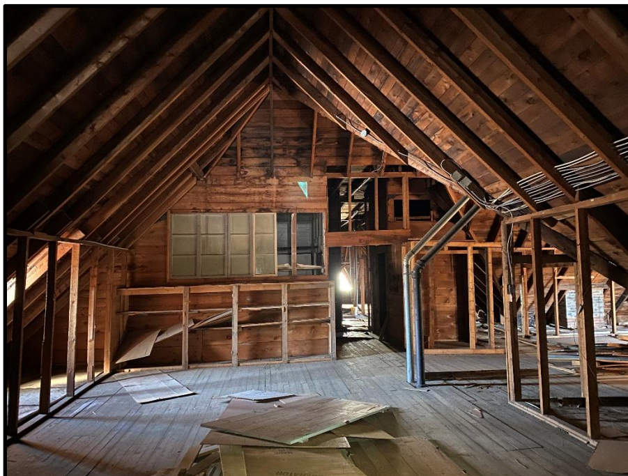
Photo 14: Attic of subject building.
