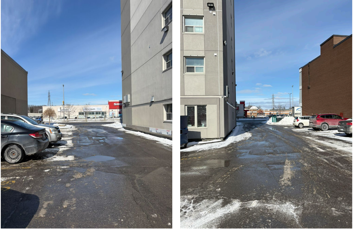
Figure 3. View of existing site access/egress on the west (left) and east (right) sides of the existing building looking towards Carling Avenue
