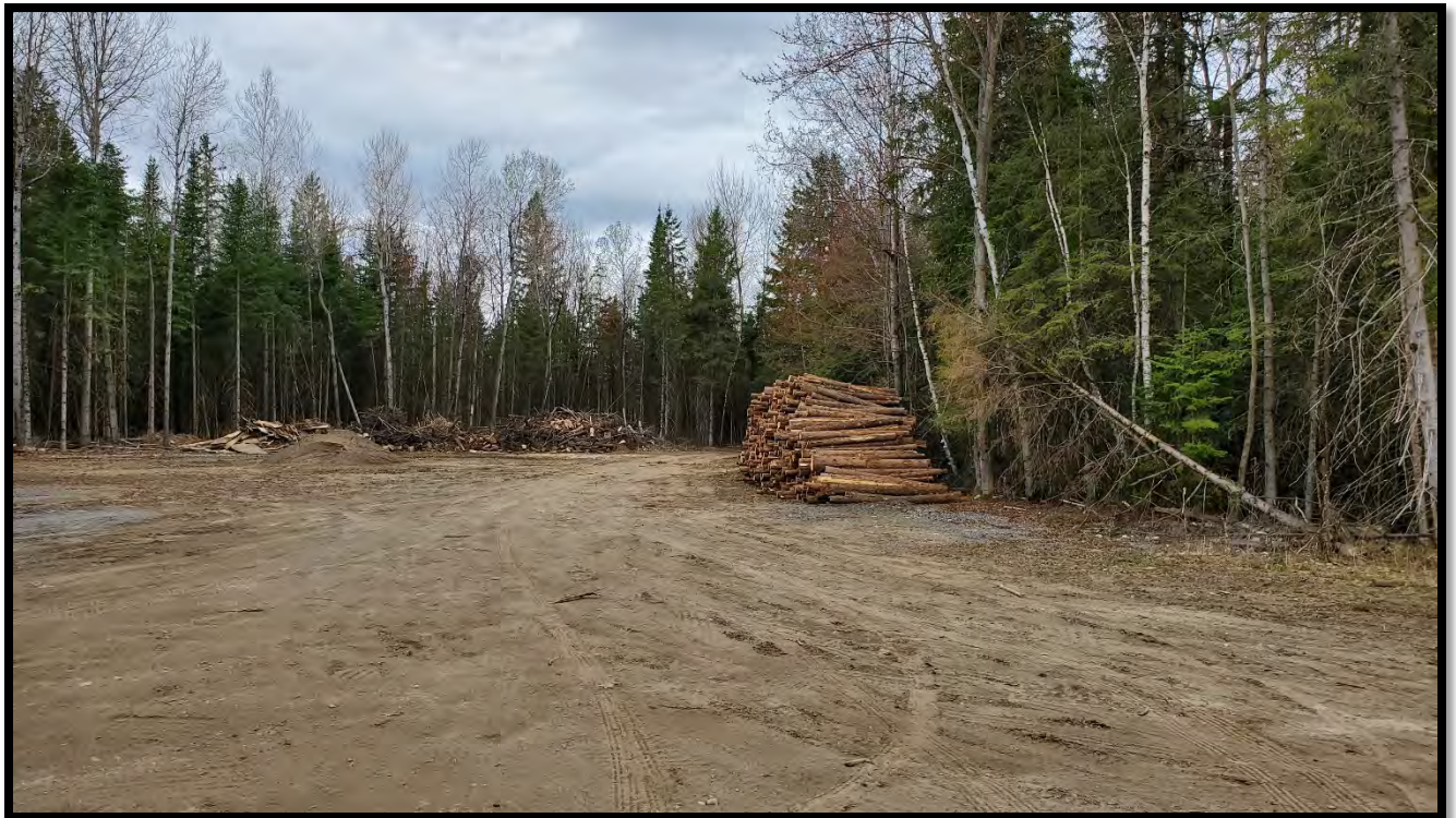
Figure 2: Cleared area off Diamondview Road (D03).
