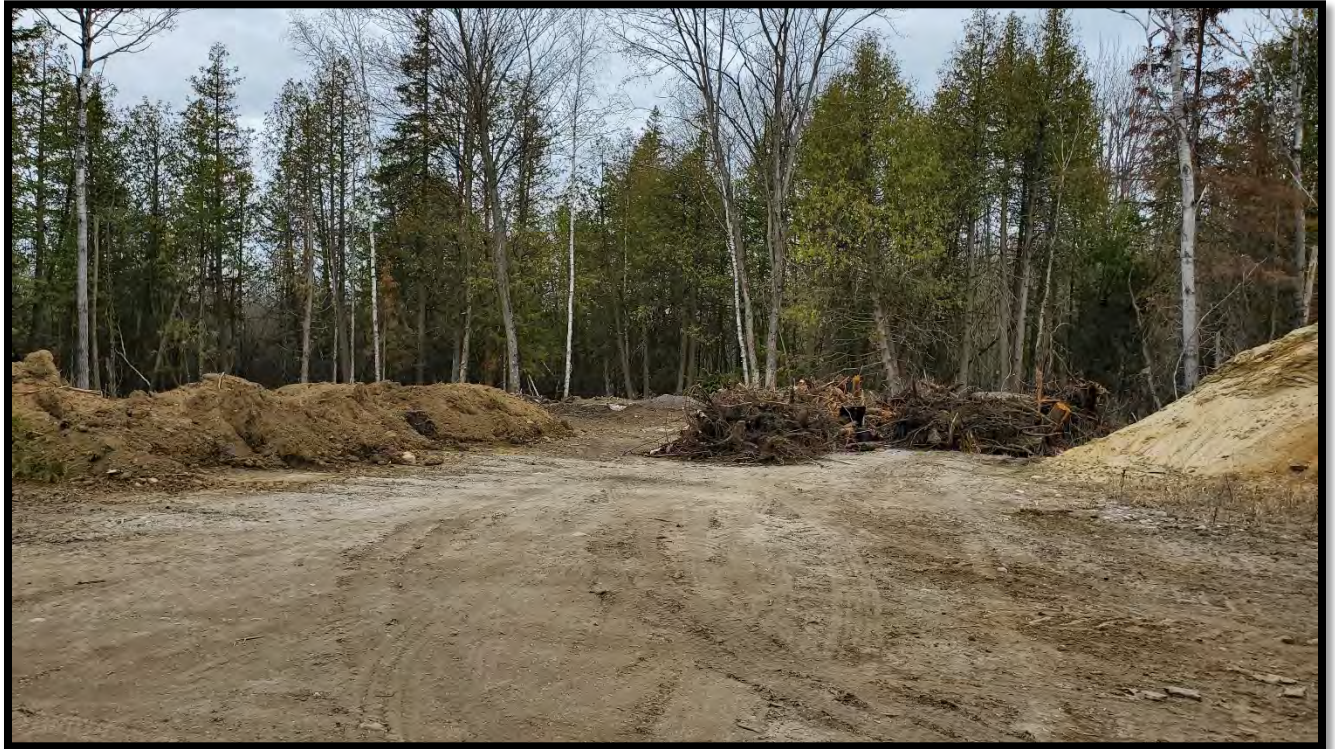
Figure 3: Cleared area off Diamondview Road (D01).
