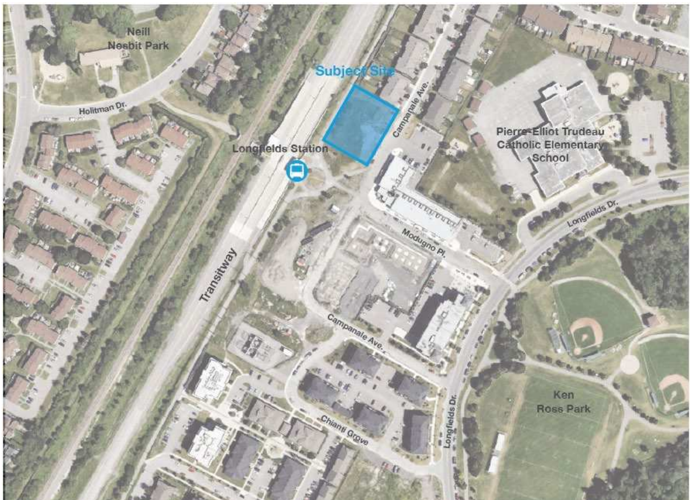
Figure 1: Aerial view of the subject site.
