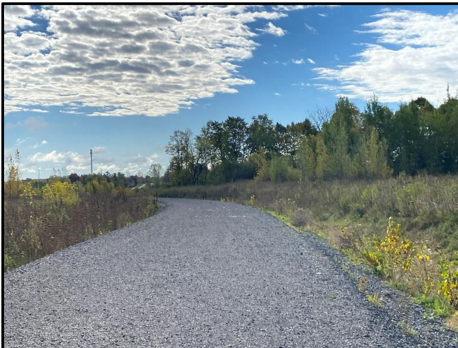
Photo 4: Construction access road on the west side of the Phase I Property, picture taken facing south.
