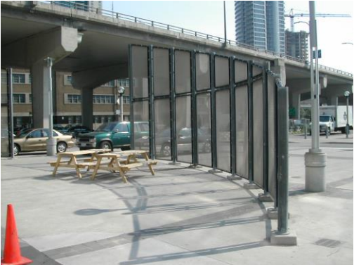
Image 12: Wind Control Examples at Grade
