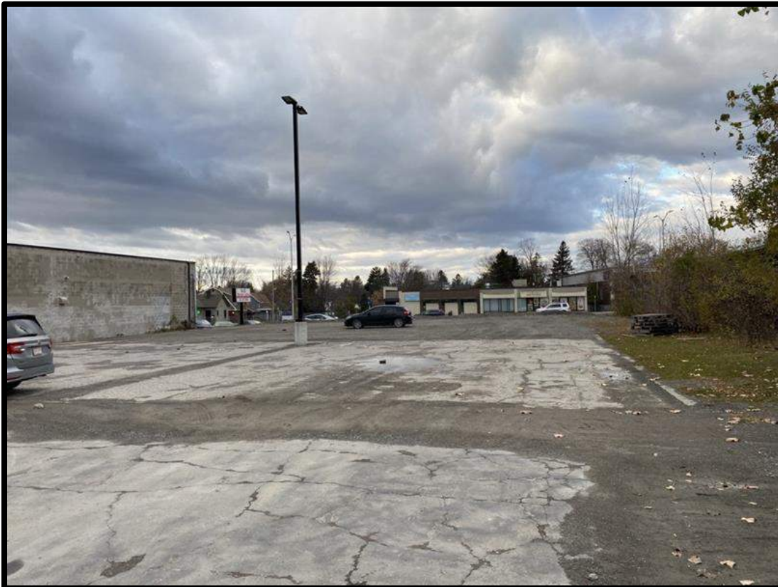
Photograph 2: View of 1746 Carling Avenue, facing north.
