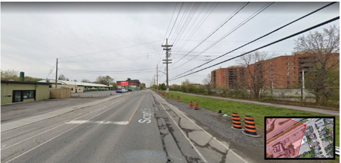
Figure 8.0 - Existing Site Conditions, View West along Scott Street.
