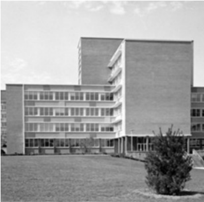
Figure 85: Sir Charles Tupper Building. Source: CLC
