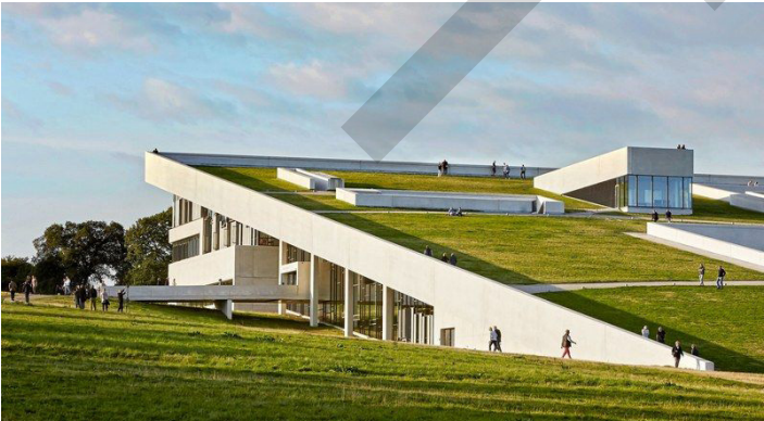
Figure 127: Green roof. Source: Henning Larsen Architects
