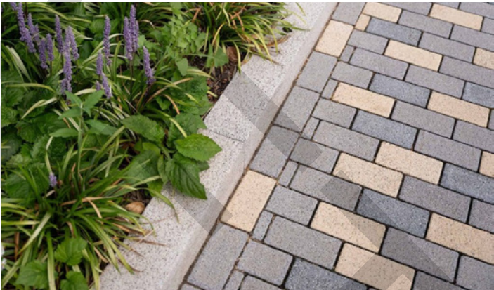
Figure 126: Permeable paving. Source: Fotenn
