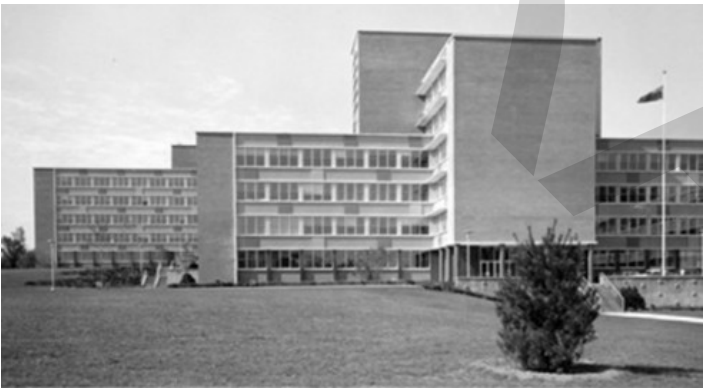
Figure 43: Sir Charles Tupper Building. Source: CLC
