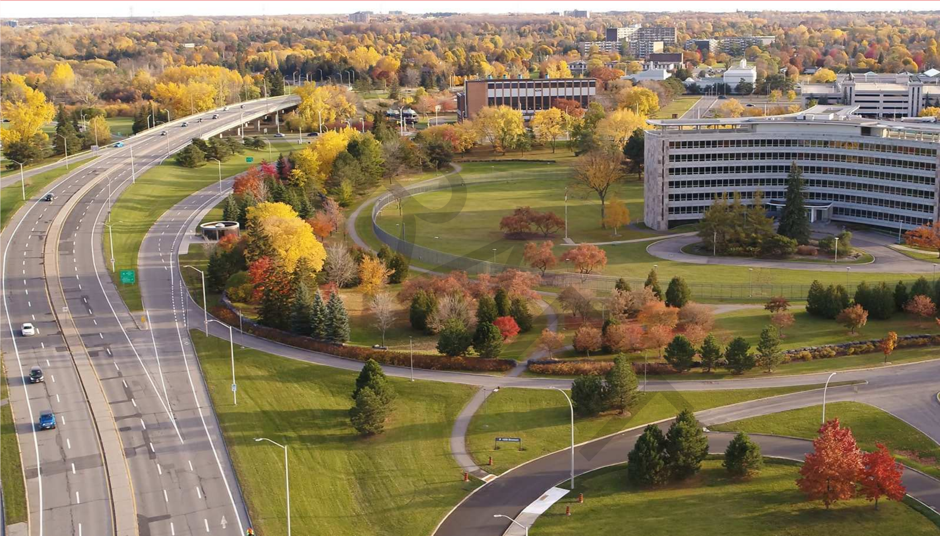
Figure 31: Bronson Ave and ramps. Source: CLC
