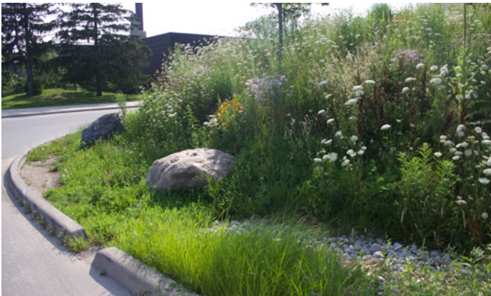
Figure 124: Bioswale. Source: Fotenn
