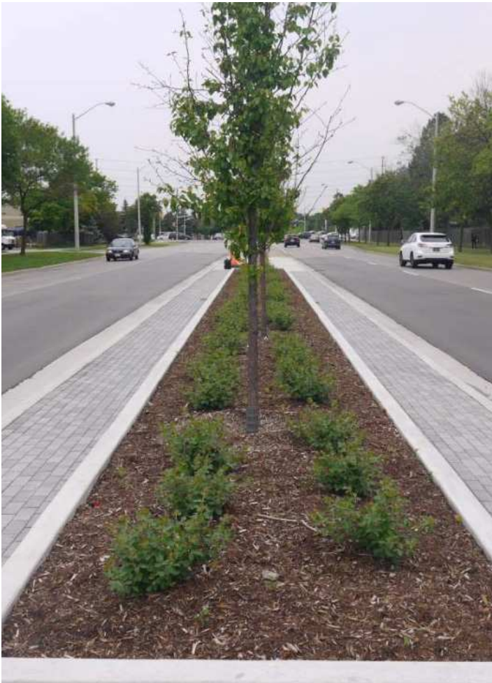
Figure 125: Stormwater tree trechnes in Mississauga, ON. Source: CVC
