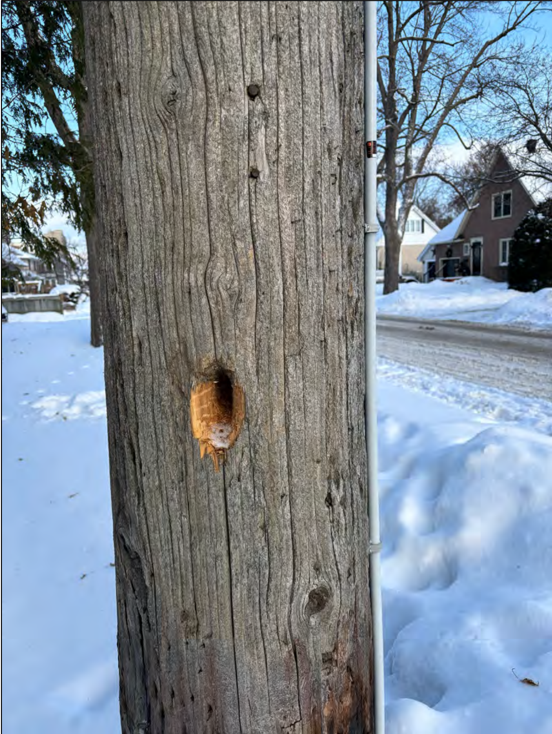
Photo 5: Hydro pole on City of Ottawa property with potential Pileated Woodpecker foraging cavity
