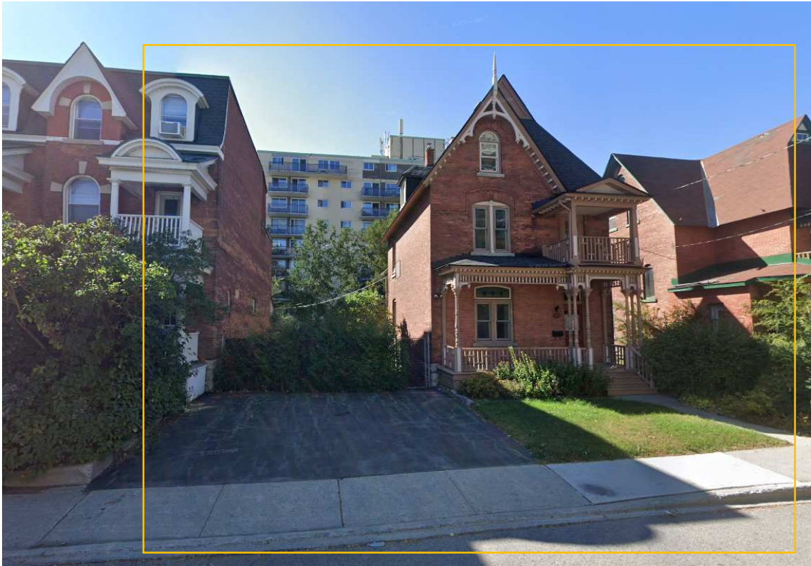
Figure 3: View of the site from Nelson Street. The directly adjacent buildings are of similar height and setback.
