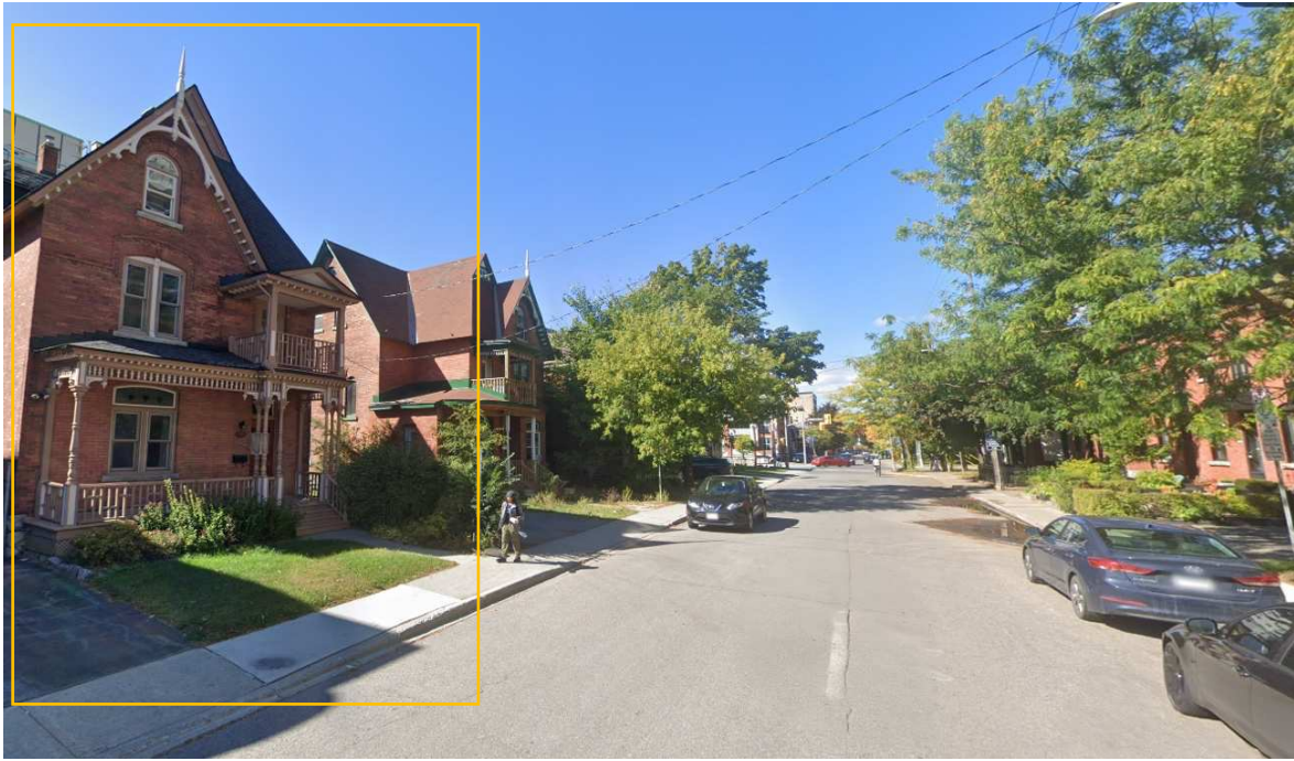
Figure 7: View of the subject property (left), looking north up Nelson Street towards Laurier Avenue
