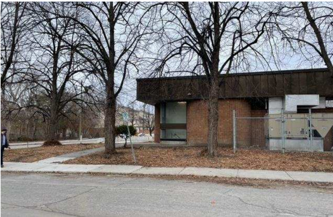
Photograph 4: View of southwestern portion of the Phase I Property.
