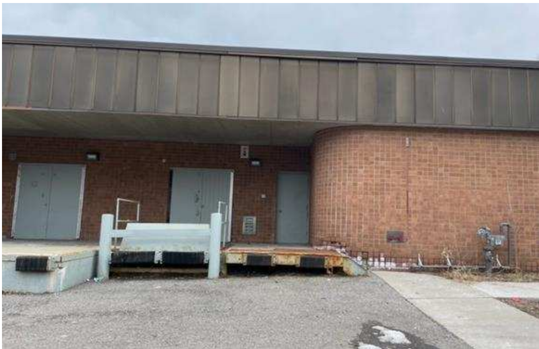
Photograph 2: View of west side of the building exterior or loading bay.
