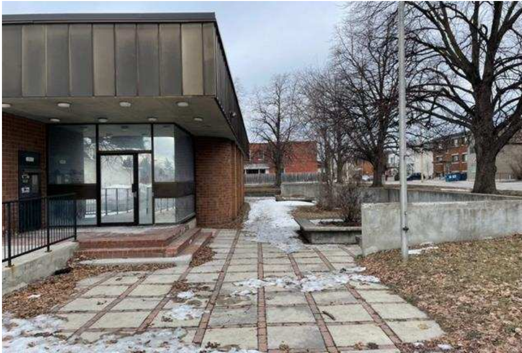
Photograph 1: View of eastern side of the Phase I Property.
