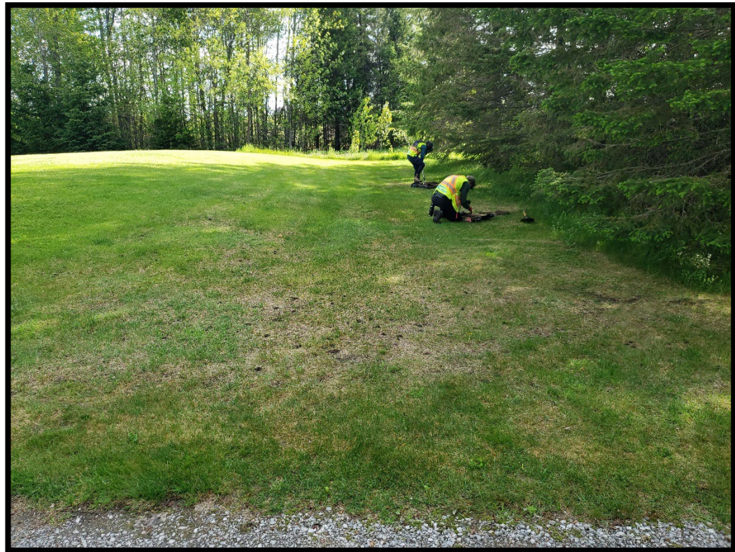
Figure 10: Test pitting in progress along the raised land of the septic bed (MH1511-D003).
